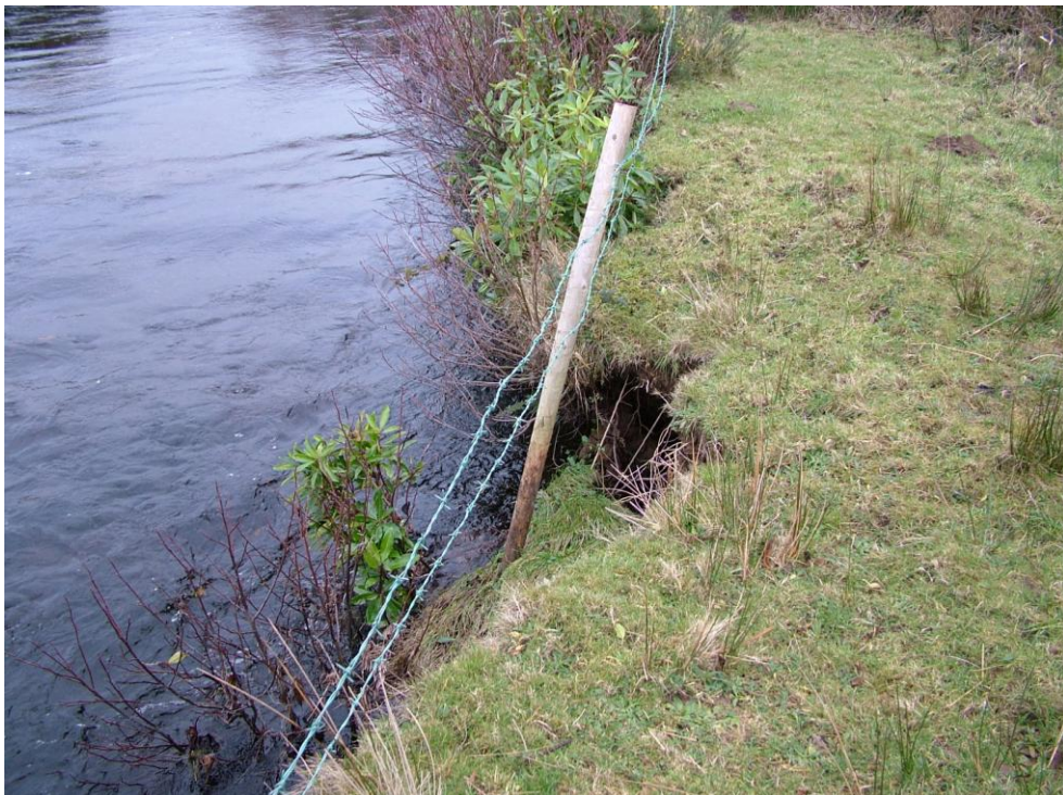
Plate 24: Fence undermined by riverbank collapses.
