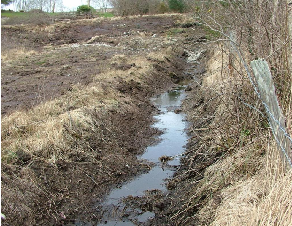
Plate 15: New drainage as part of land improvement works.
