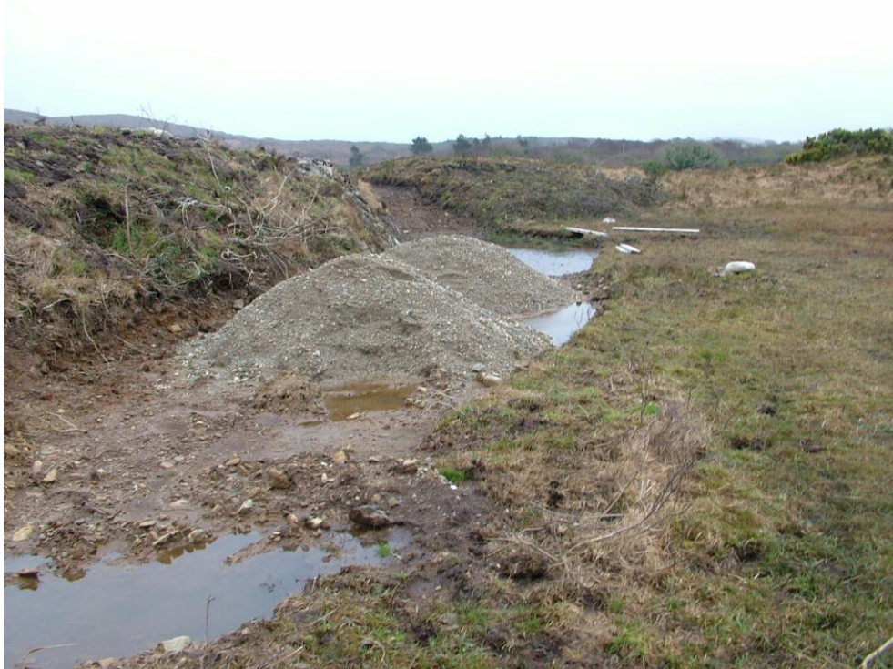
Plate 12: Construction of unmetalled roadway in blanket bog habitat.
