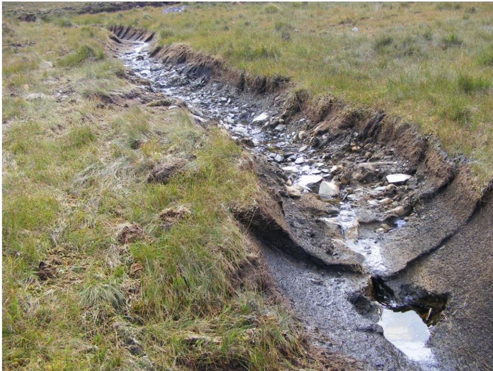
Plate 28: New drain dug on wet heath, possible candidate for blocking with a series of simple dams or peat plugs.
