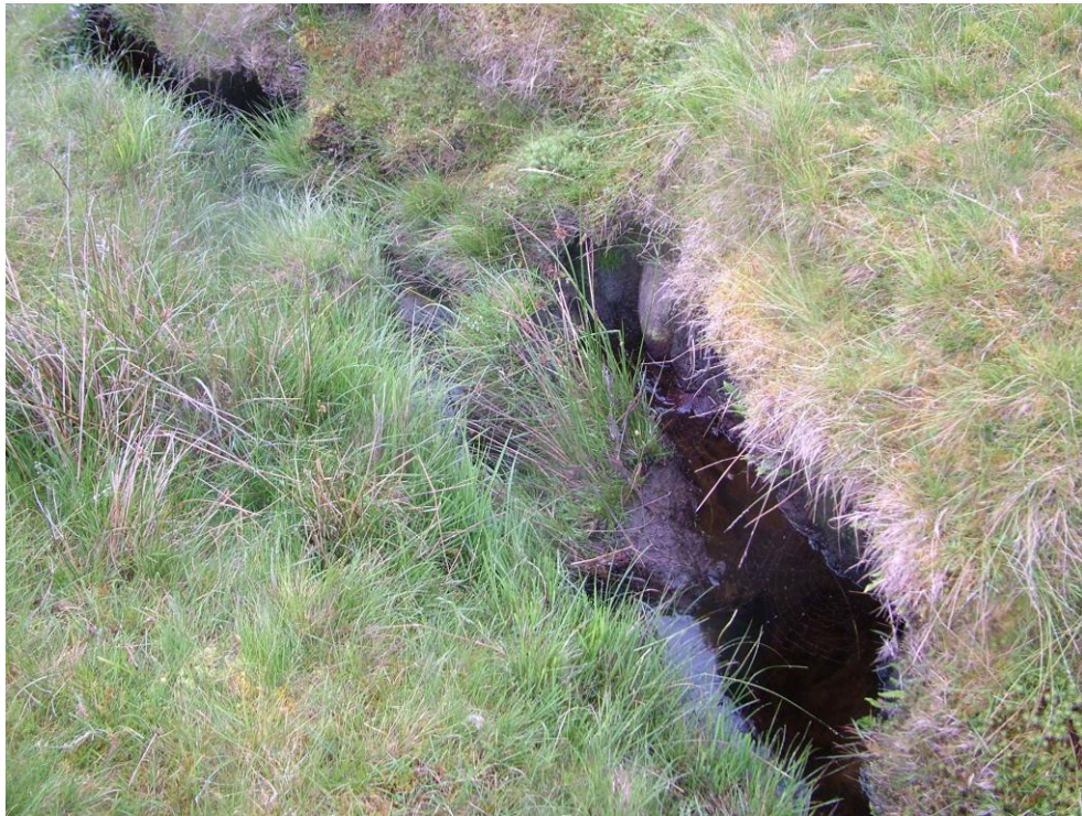
Plate 19: Collapse of the side of a drainage channel.
