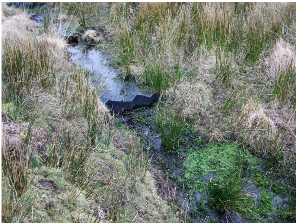
Plate 27: Simple plastic dam, Note the establishment of Sphagnum spp upstream of the blockage.
