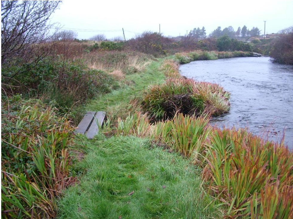
Plate 37: Simple bridges to prevent damage from pedestrian traffic at points where minor watercourses enter the main channel.
