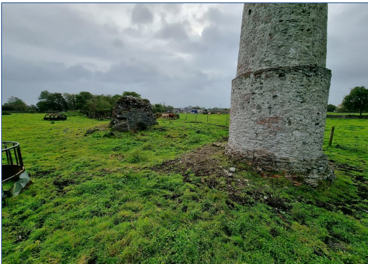
Figure 2 View across the site.
