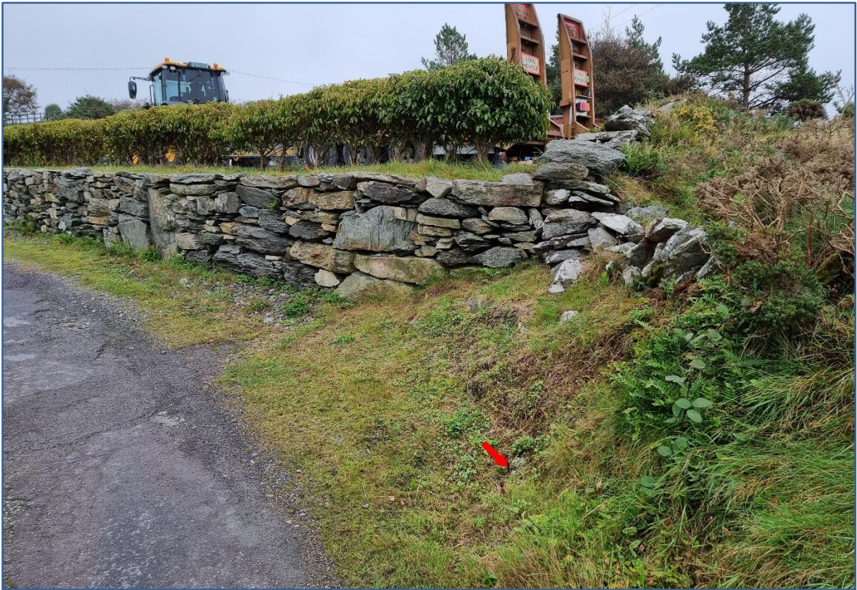
Figure 2 Location of Cephaloziella nicholsonii , at the base of an old roadside retaining wall.
