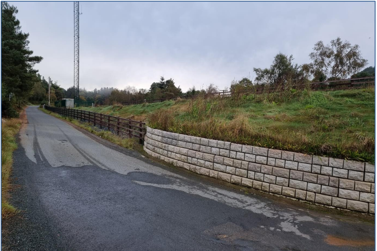
Figure 2 Railway bank that supported Calaminarian grassland in 2018, but has since been lost due to its capping with inert soil.
