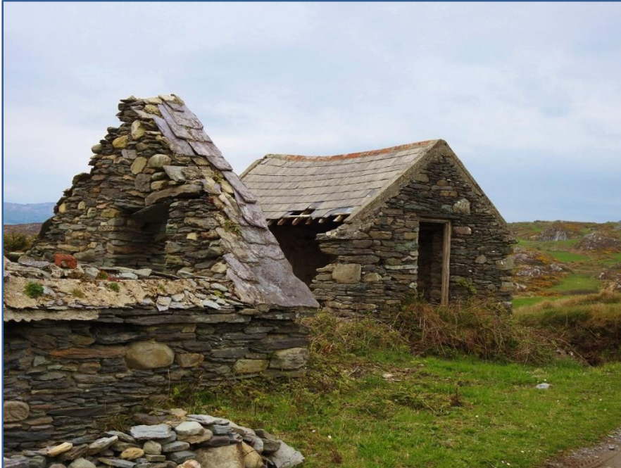
Figure 15 Old homesteads such as these near Mizen Head (Co. Cork) make suitable nest sites for Chough, especially where part of the roof is intact. Photograph © Declan O'Donnell, NPWS.
