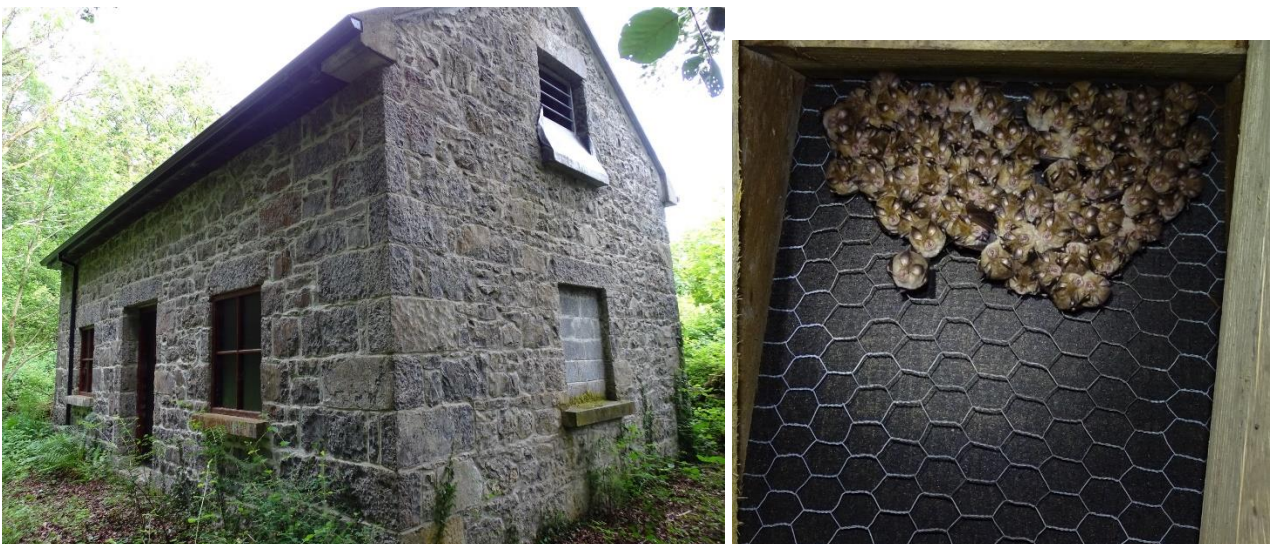
Plate 1a,b: Garryland Lodge (external view) and Lesser horseshoe bats in roof space (internal).
