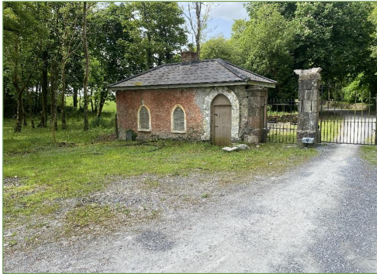
A7. View of the southern gate lodge that does not house the maternity colony of Lesser Horseshoe Bat.
