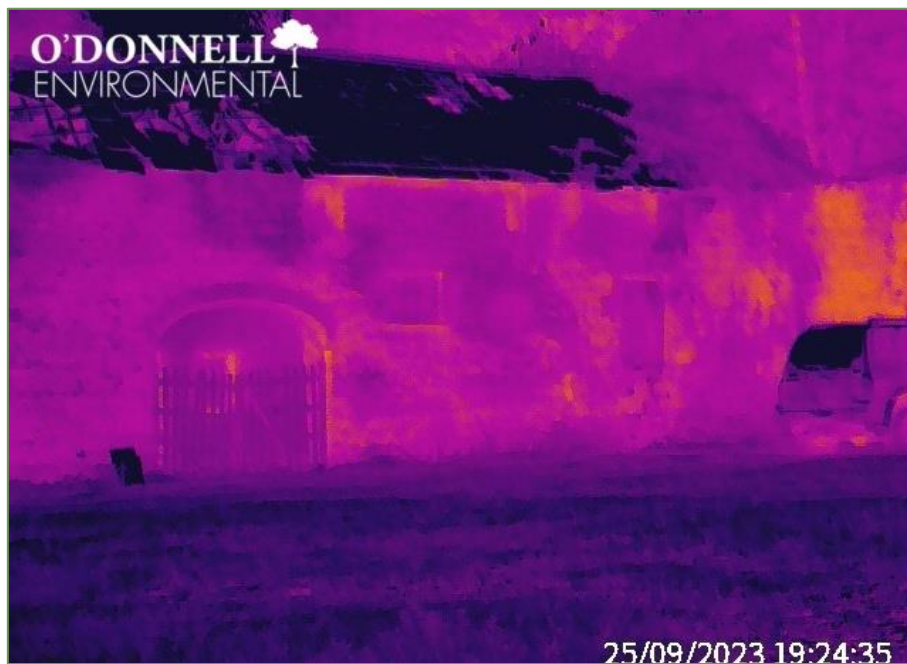
Plate 2.7 Example image of thermal camera covering the eastern aspect of the two-storey outbuilding adjoining the eastern courtyard
