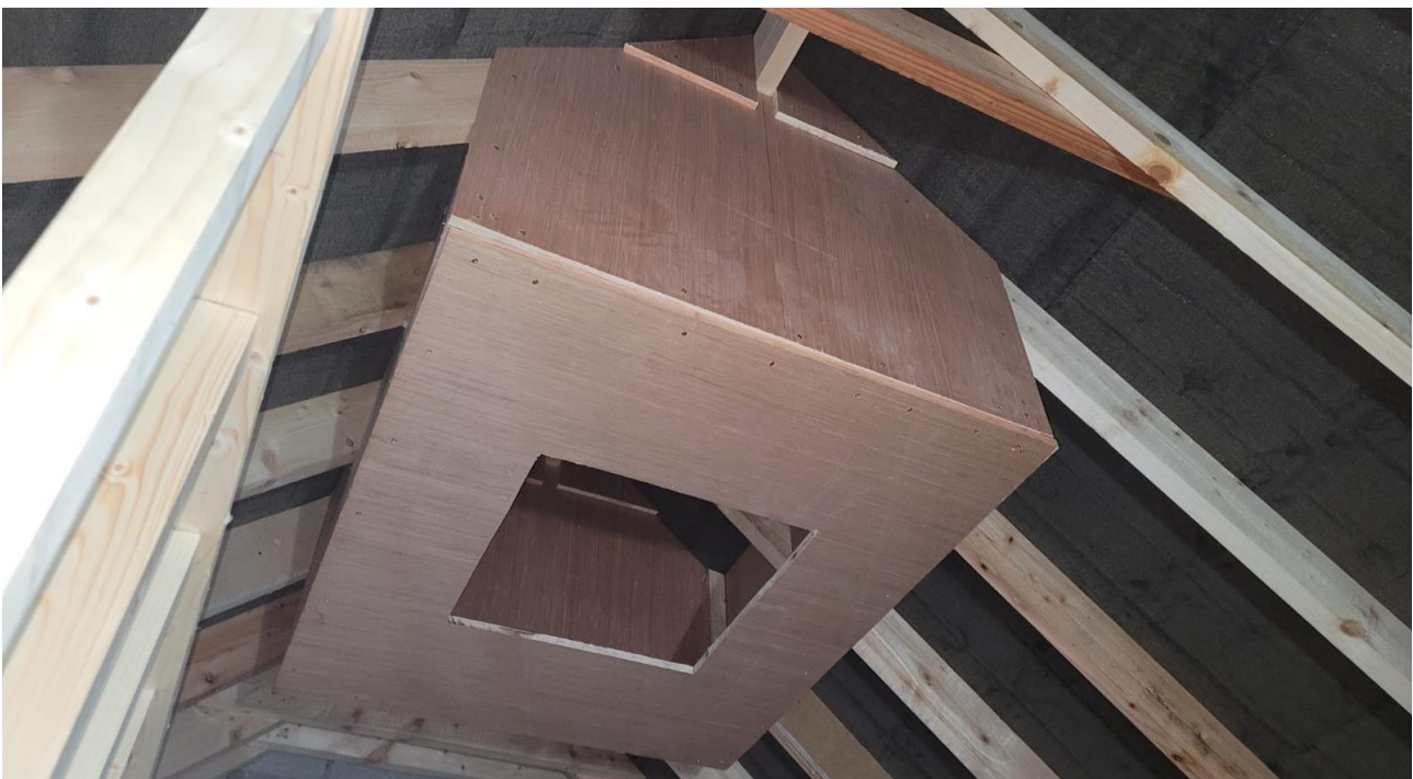
Plate 3a: Hot box installed in roof of bat house.
