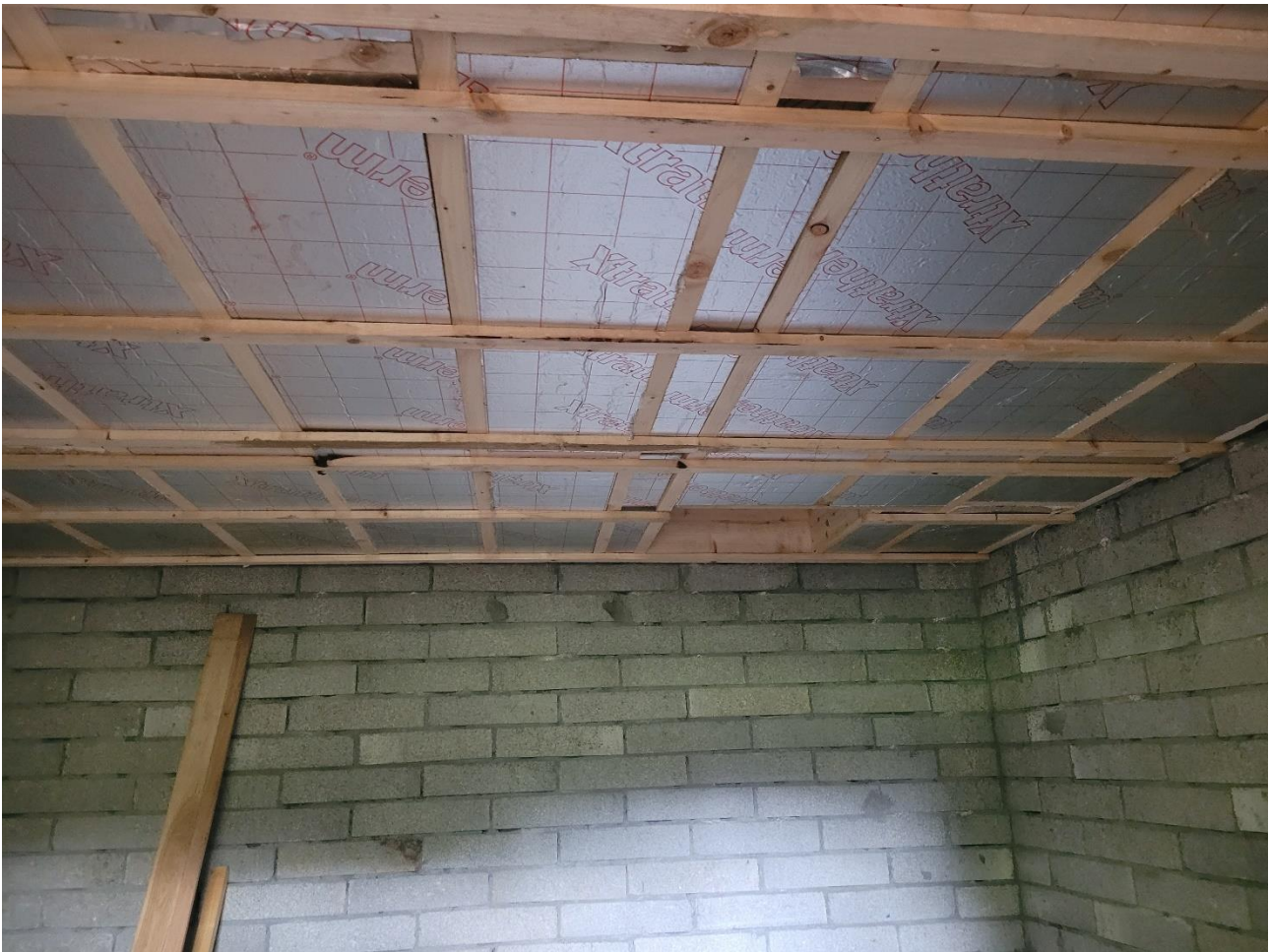
Plate 4: New insulated loft floor – showing underside of loft floor.
