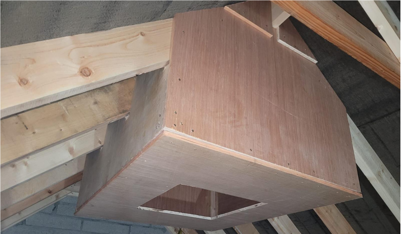
Plate 3b: Hot box installed in roof of bat house.
