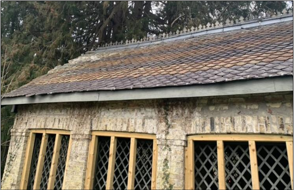
Plate 3-1: Slated roof structure on the Boathouse (photo taken 13 th February 2023)
