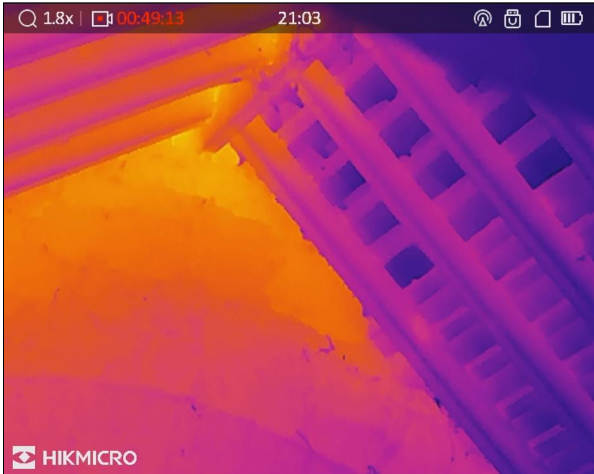
Plate 2-5: NVA viewshed of roof and wall inside the Boathouse
