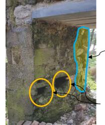
Window reveals to be consolidated and repointed were required. New salvaged stone to match the existing to be keyed in were required.
