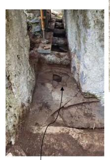
Allow for the vegetation to be moved and the existing drainage stones to be repointed. Allow for 1 number new curved stones across the joints in the wall walk. Drainage stone is to be bedded in lime mortar, refer to Architect for detail of new curved stones. Note photo from the north east corner.
