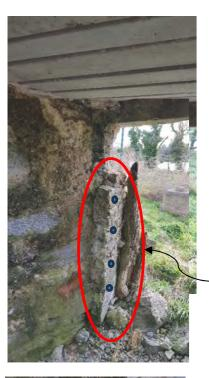
Localised rebuilding at the end of the new lintel with new / salvaged stone in lime mortar.
