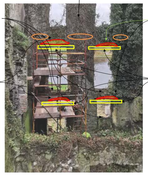
Allow for new carved stone cill bedded in lime mortar.
