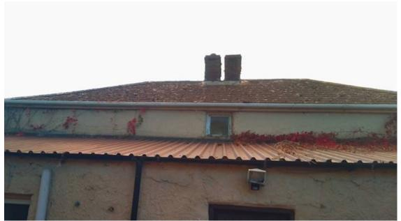
These chimneys are structurally compromised while the rest of the house did not seem to provide access to the roof or interior of the house.
