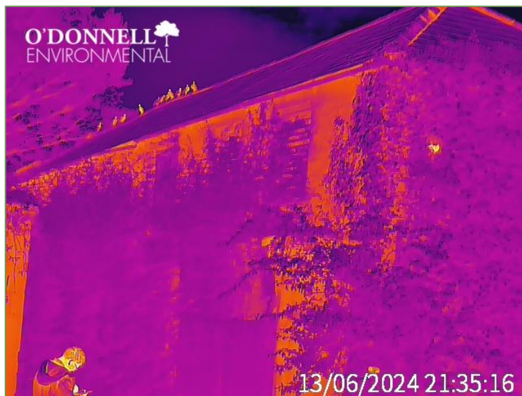
Plate 2.2 Viewshed of thermal camera and surveyor covering the front/southeastern aspect of Lissardagh Coach House(Feral Pigeons on the roof).
