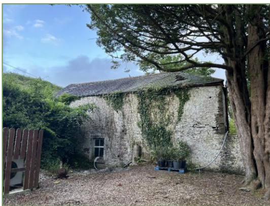
Plate 3.2.3 View overlooking the western aspect of the Coach House.
