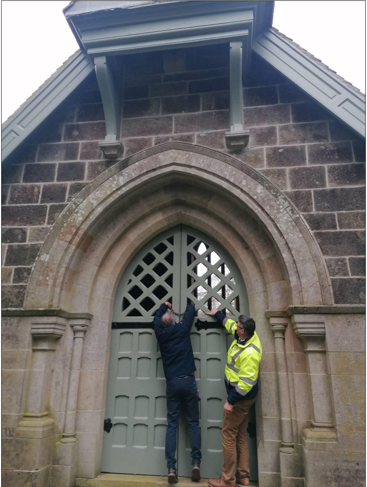
Plate 24. A lock is to be provided on the door, which is currently locked with a chain and padlock.
