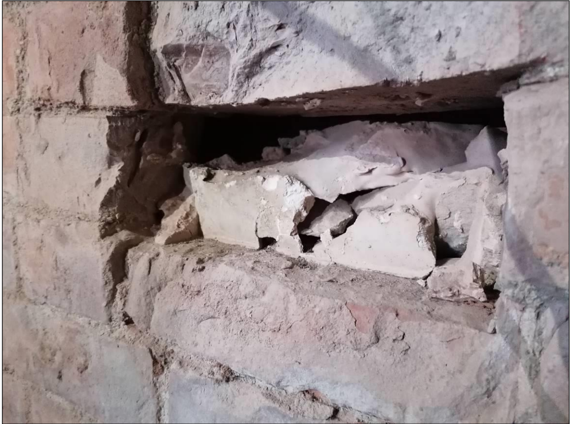
Plate 22. Potential hibernation location in the brick work – to be retained.
