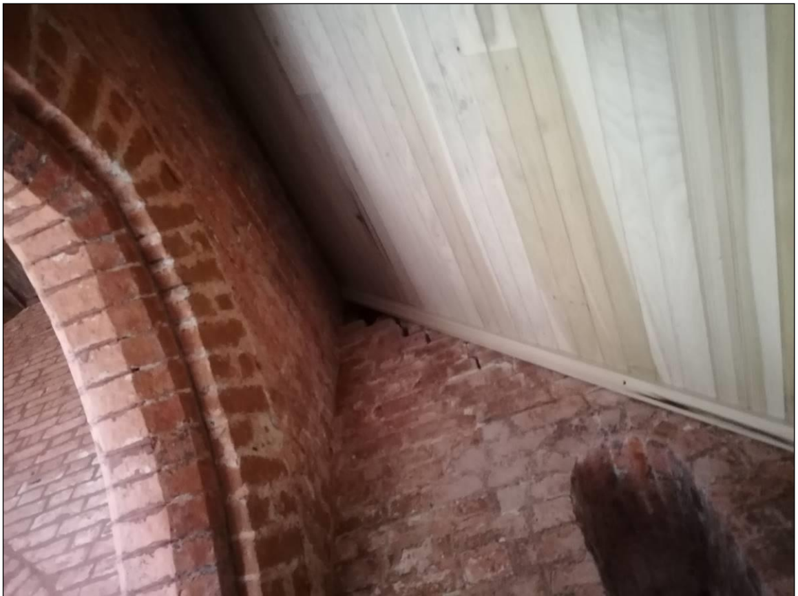
Plate 19. Newly installed tg&v sheeting in the aisles of mausoleum.
