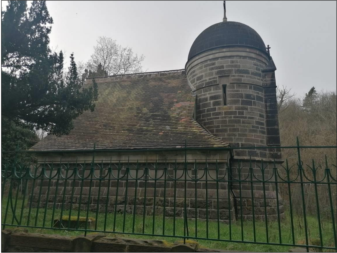
Plate 13. Rossmore Mausoleum in December 2023 – note repaired clay tiles on the roof.
