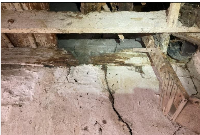
Plate 9 Gap in ground floor ceiling to attic space - note bat and bird droppings on wall (2023 surveys).
