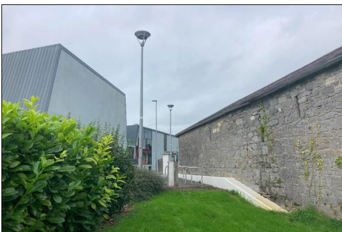
Plate 5 Side of building adjacent to playground with adjacent street lighting
