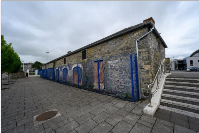
Plate 1 The subject building in Thurles, Co Tipperary, July 2024.
