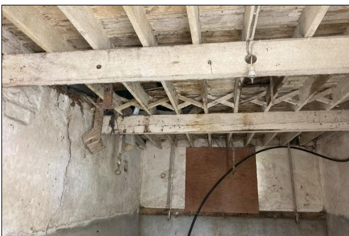
Plate 6 Interior space below attic (2023 surveys).
