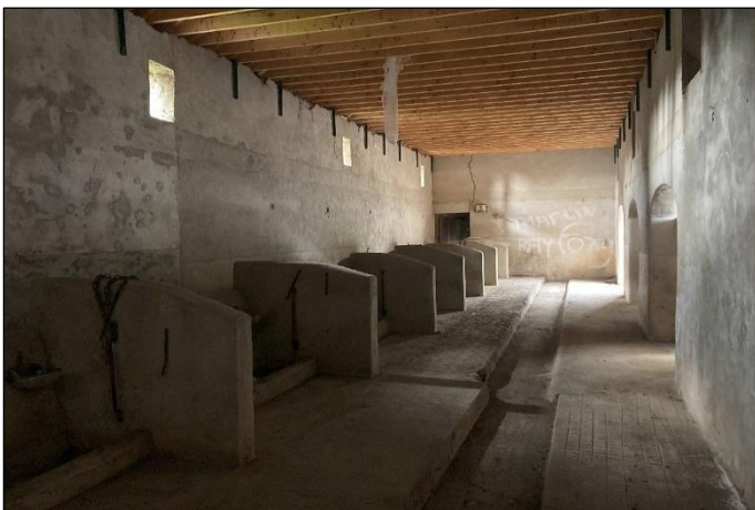
Plate 8 Main central livestock feeding hall - note new timbers (2023 surveys).
