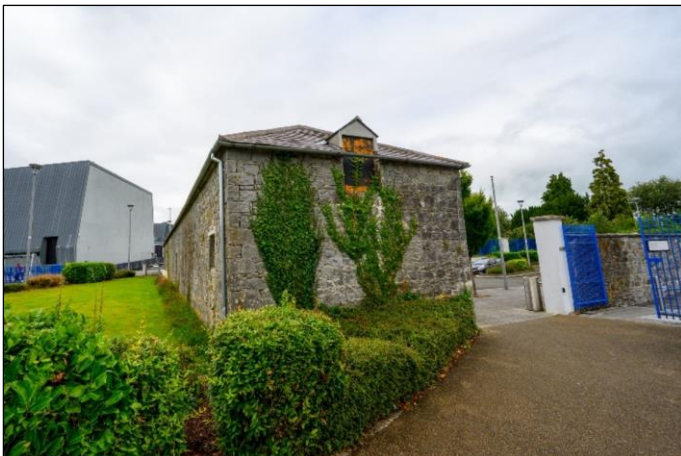
Plate 2 The subject building in Thurles, Co Tipperary, July 2024.
