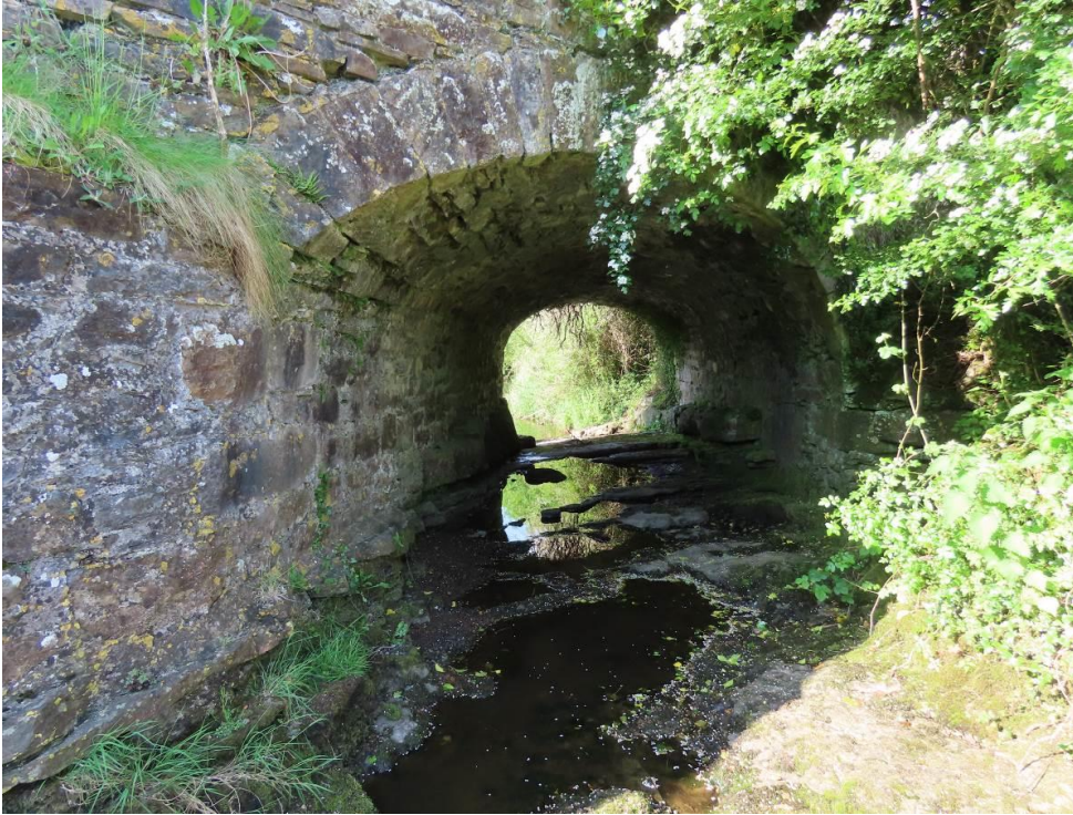
Photo 5 – view under western arch – practically dry on date of survey
