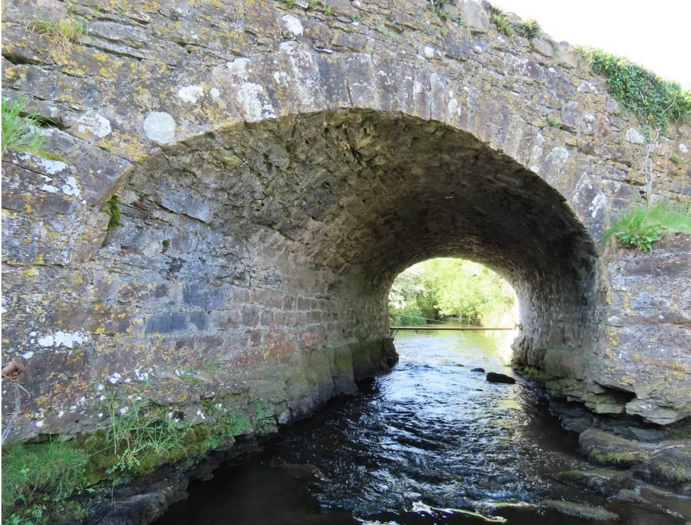
Photo 11 – view under middle arch from upstream
