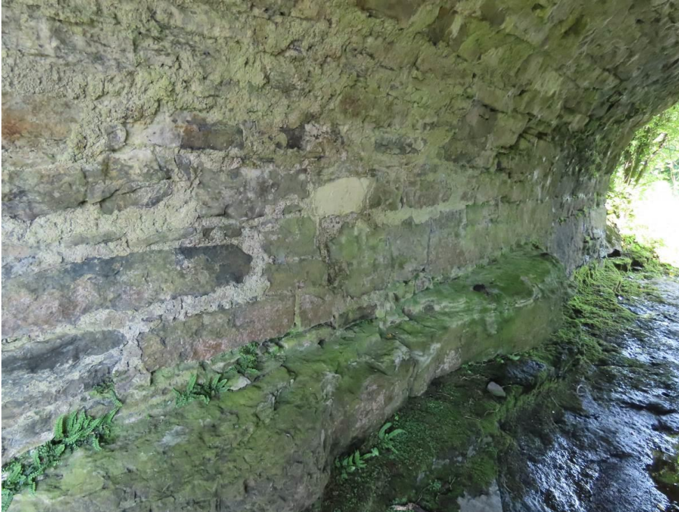
Photo 9 – stone plinth under westernmost arch
