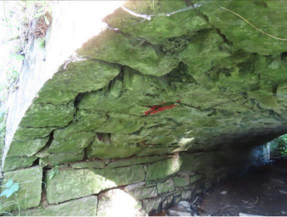
Photo 47 – crevice marked for retention
