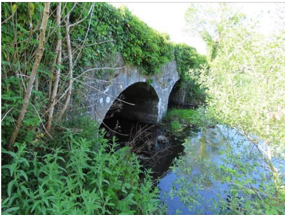
Photo 42 – view across downstream face of arch
