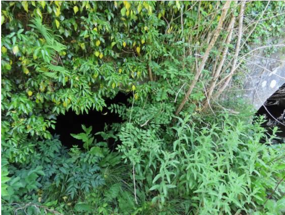
Photo 41 – westernmost arch obscured by vegetation
