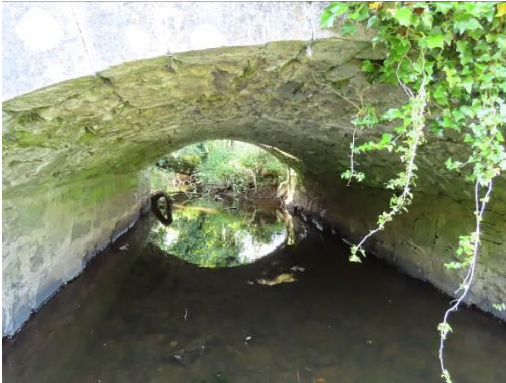
Photo 43 – view under arch 1
