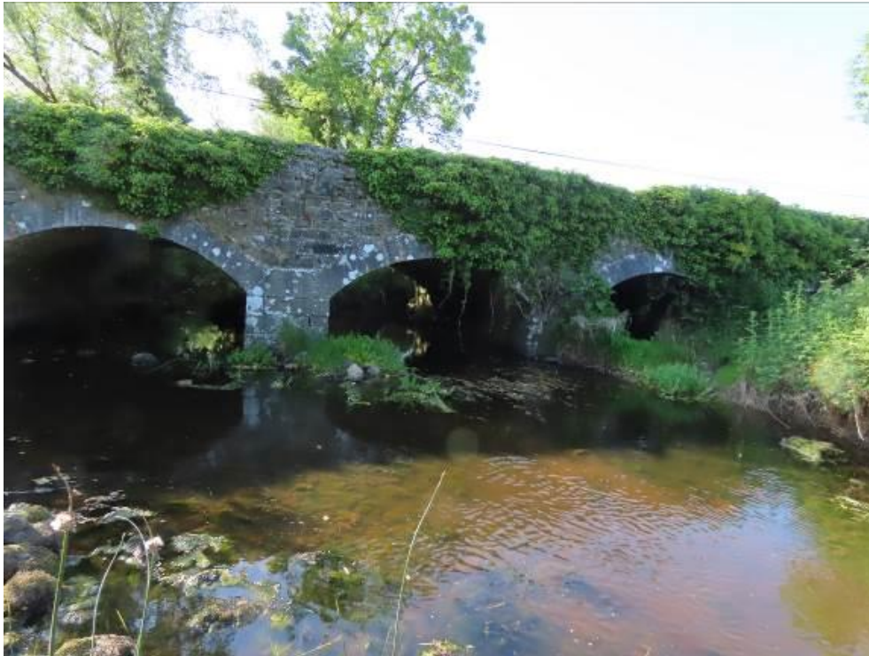
Photo 51 – downstream elevation of bridge
