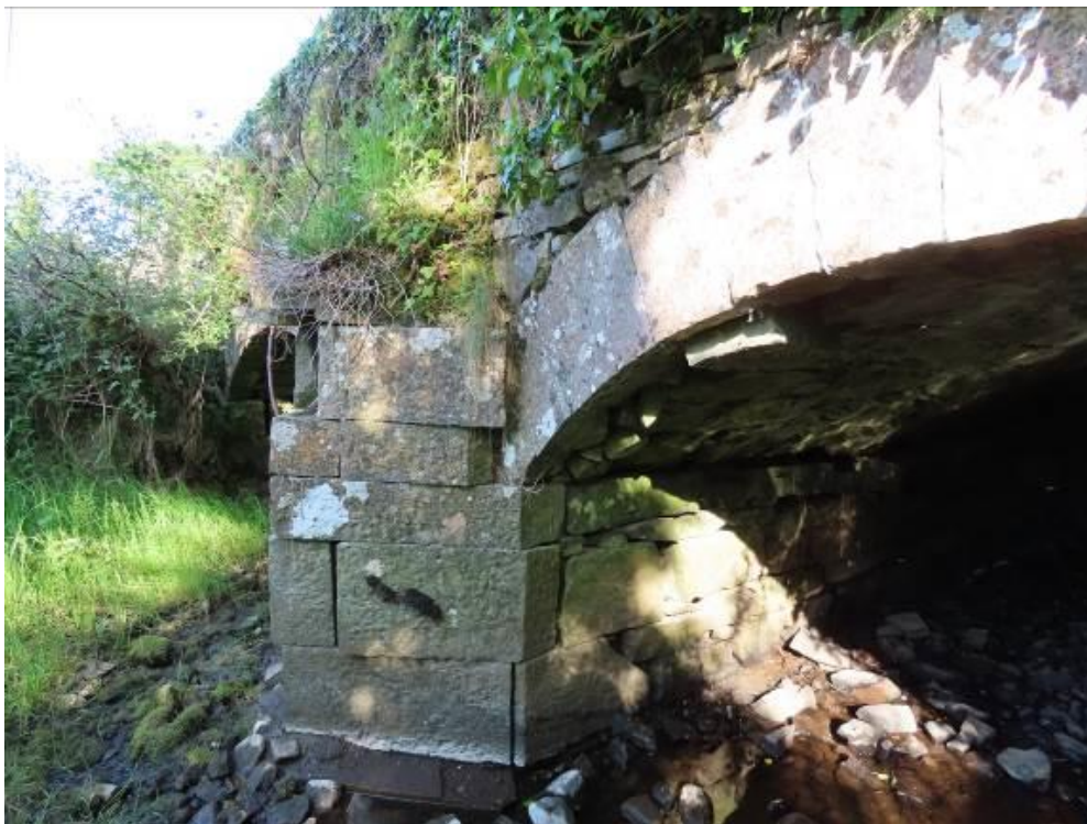
Photo 46 – damaged pier
