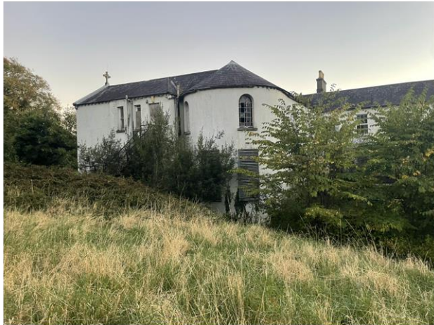
Plate 4: View of sloping ground to the north of the convent building
