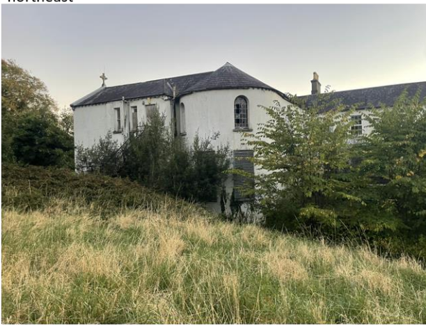
Plate 4: View of sloping ground to the north of the convent building
