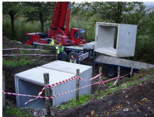
Plate 6.2: View of Flahive Hibernaculum under construction
