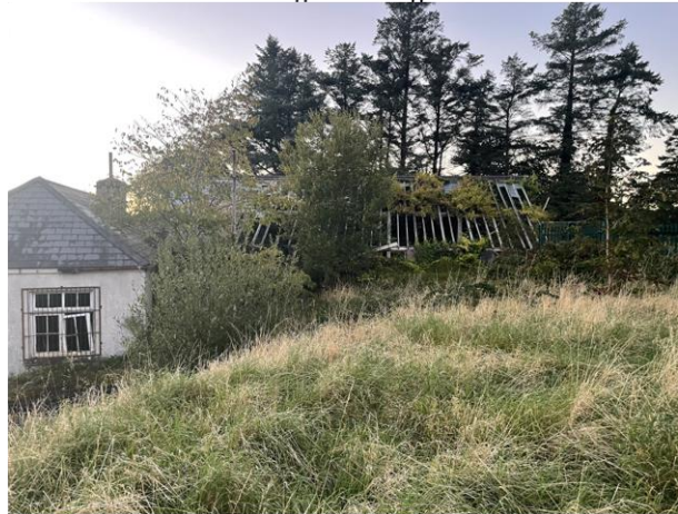
Plate 5: View of west to old kitchen and delapidated glass house
