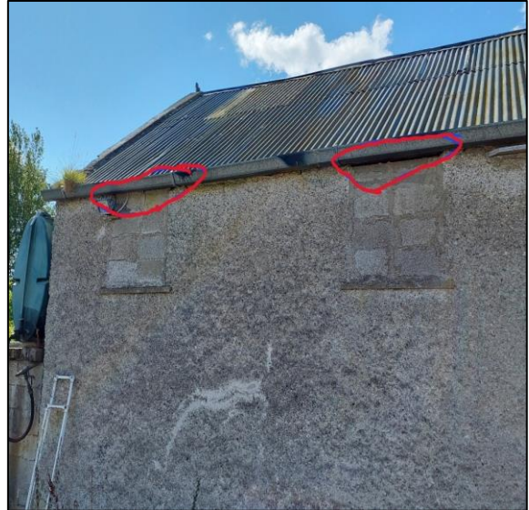
Plate 44: Cavities above former windows provide PRFs in east-facing side of S16
