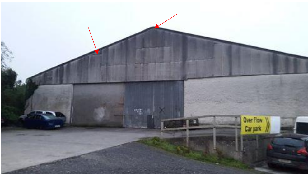
Roost areas building 3
