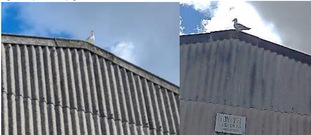
Herring gull defending a number of roofs including Building 2 and Building 7
