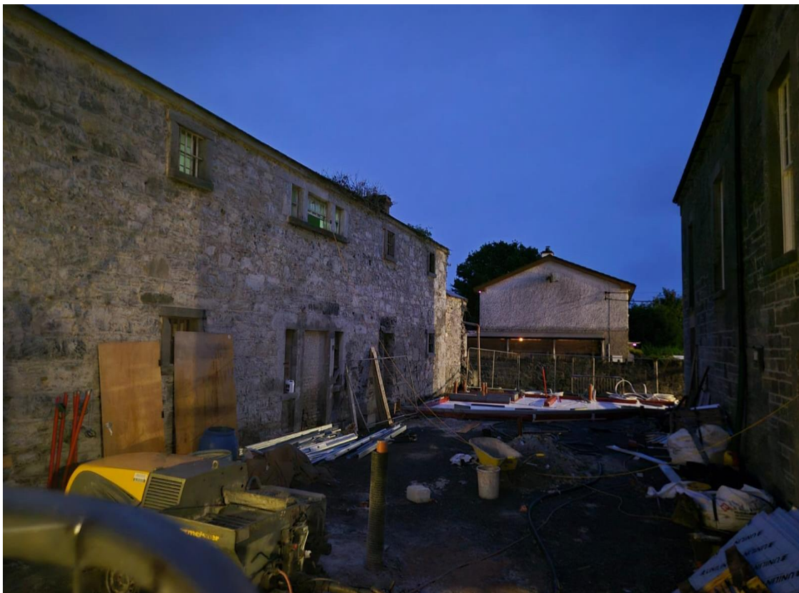
Plate 3-2: Front face in opposite direction showing light exposure from the street
