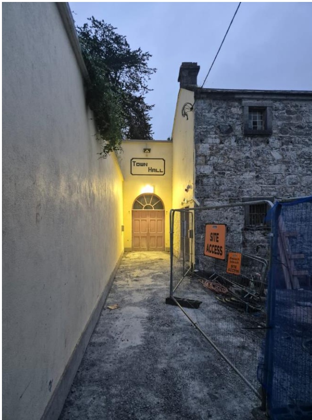
Plate 3-3: Alley next to the building with warm light above entrance
