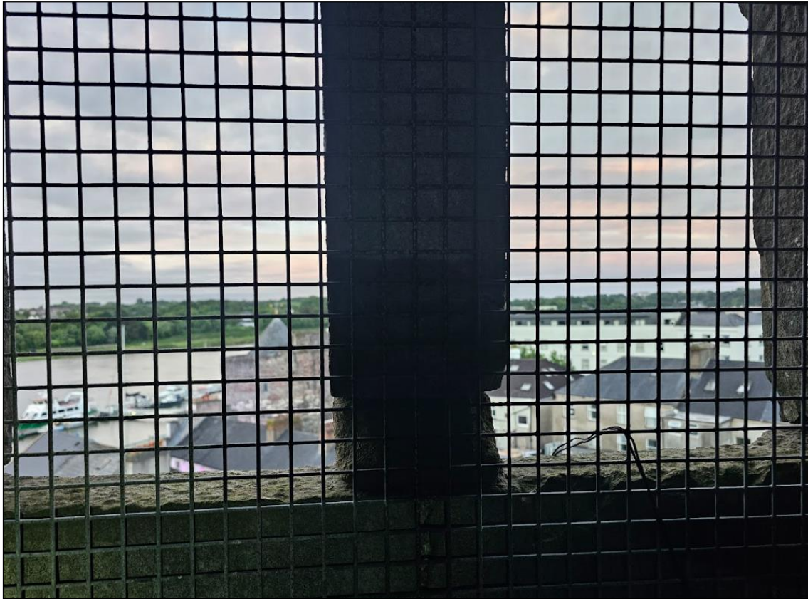
Plate 16. Removing a single row or creating an access space within the grating at the top of each of the windows will provide bat egress to the tower, without allowing other larger animals and birds such as pigeon to enter.
