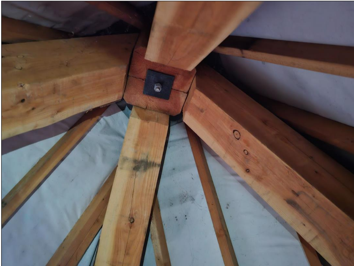
Plate 18. Level 3, Attic of the tower. By covering the roofing membrane with rough wood panels, the risk of entanglement in these roosting areas can be reduced.
