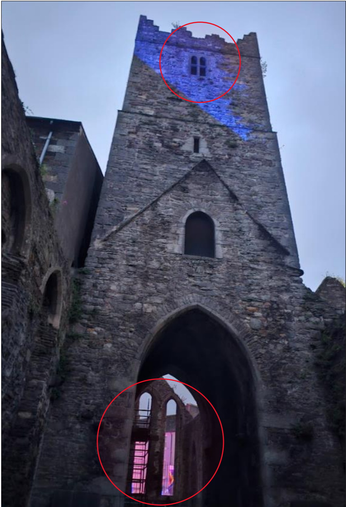
Plate 13. Light pollution from neighbouring properties shows at ground level and at the roost exit on Level 3 of the tower, circled in red.
