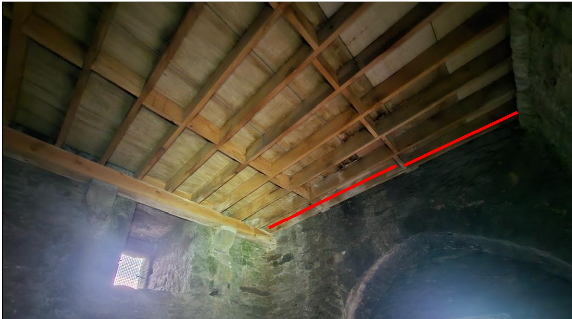
Plate 17. Level XX, showing a covered ceiling with exposed joists. This provides safe roosting opportunities for bats, without risk of entanglement in roofing membranes. Timbers here can be doubled up to create a roosting location for bats – indicative locations for timbers shown by red line.
