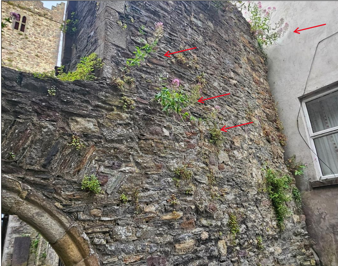
Plate 20. Examples of Red Valerian growing on the perimeter walls of the entrance to the French Church (circled in red).
