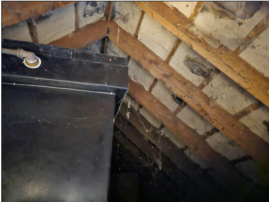
Plate 12. The water tank in the attic above the Office/File Storage/Games Room.
