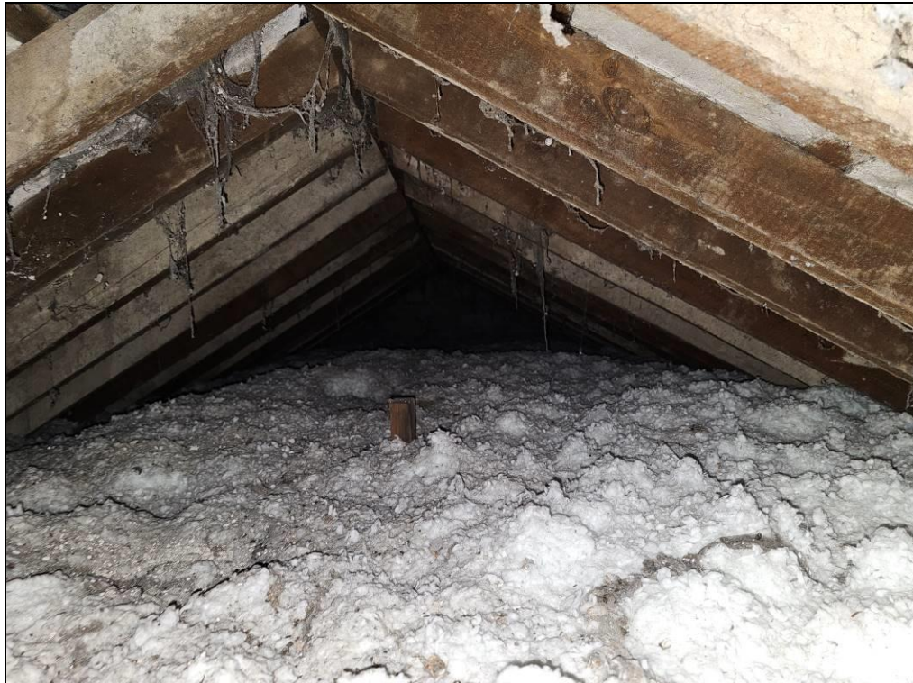
Plate 1. The attic of the main house.
