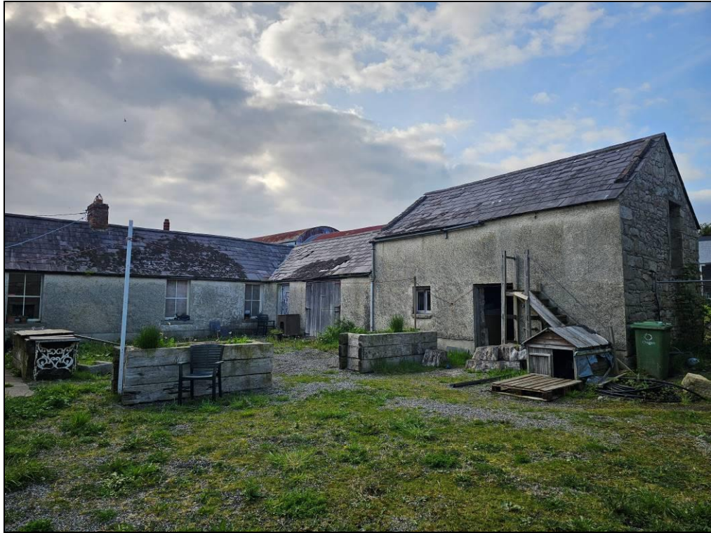
Plate 3. The 'Dog Shed', the 'Wood Shed' and the former dairy 'Store'.
