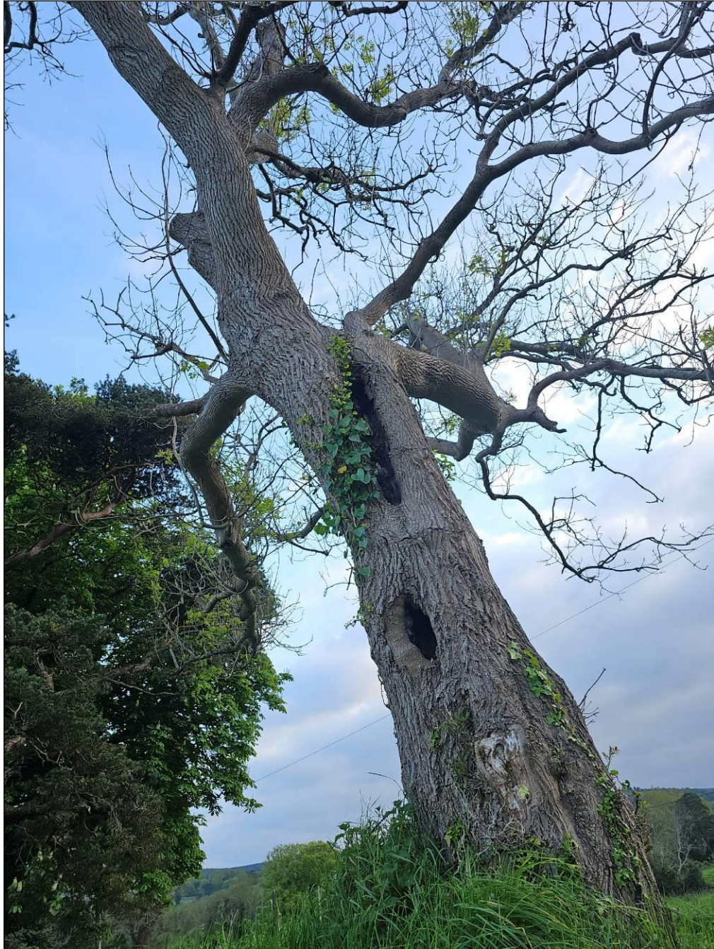
Plate 14. Ash tree with large cavities offering bats roosting potential on the drive.
