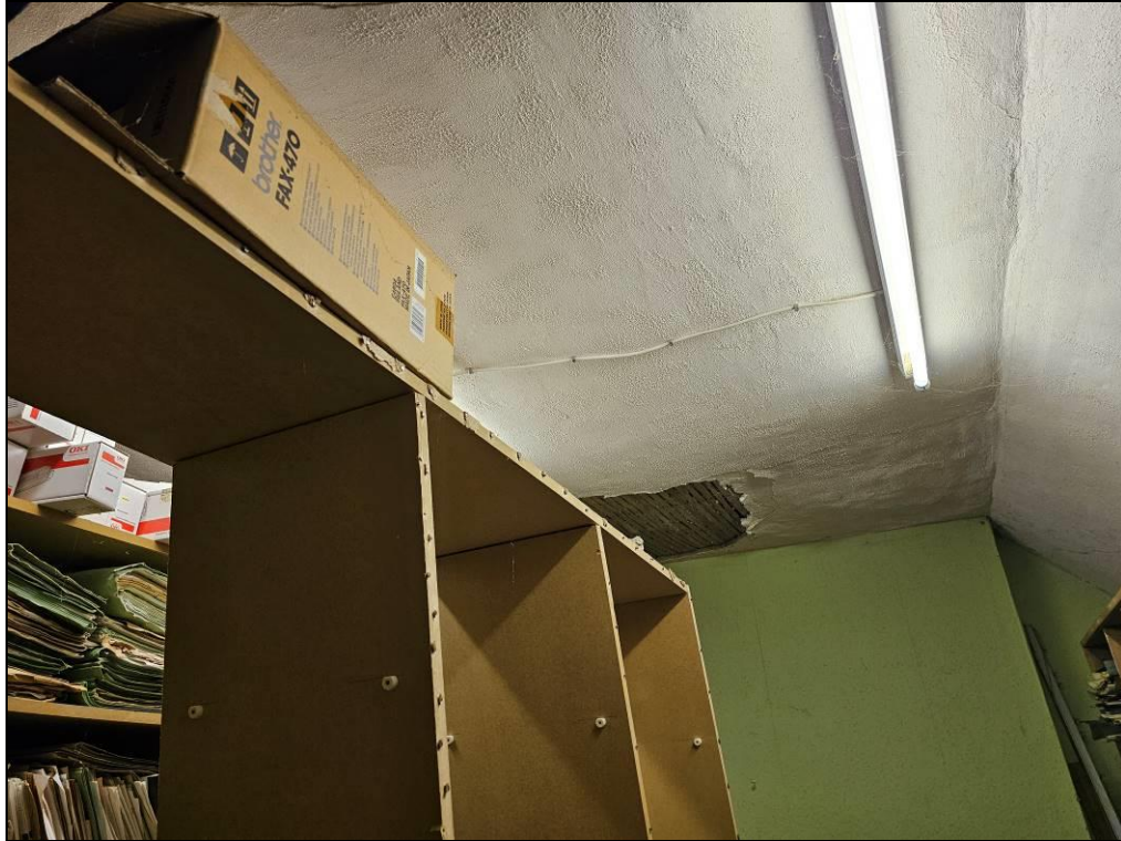
Plate 13. Traditional lathes with plaster on the ceiling of the 'File Storage Room'.
