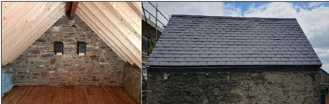
Plate 3: Internal area of dedicated bat roosting loft showing rafter roost crevice timbers & bat boxes (left) and western roof slope with 2 x bat access slates (right).
