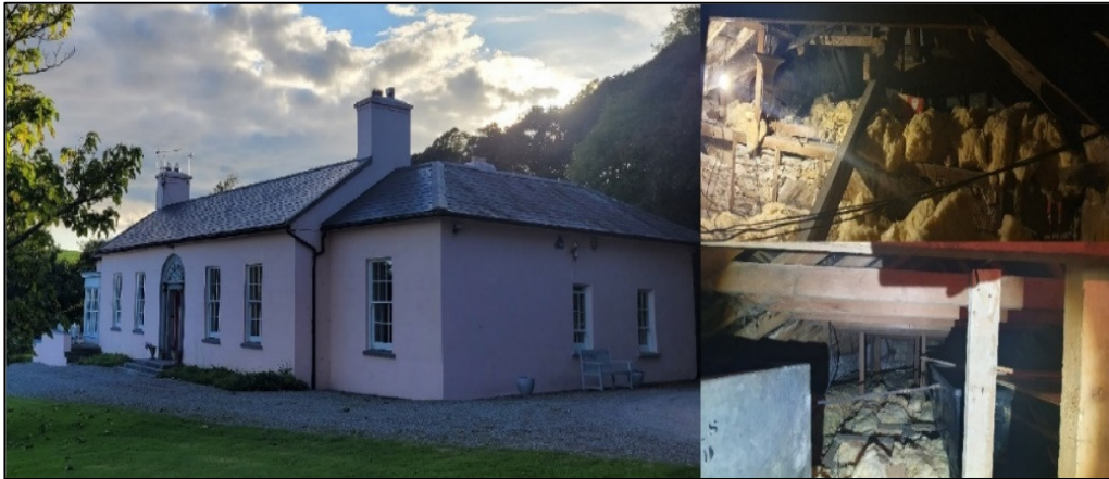
Plate 2: Sprayfield House dwelling (left) and internal attic spaces (top & bottom right).
