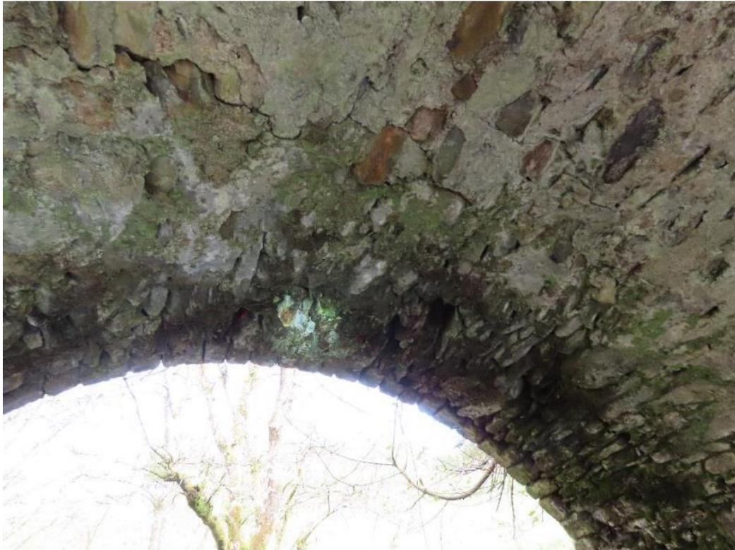
Photo 9 – fissure running around arch barrel close to downstream face of eastern arch
