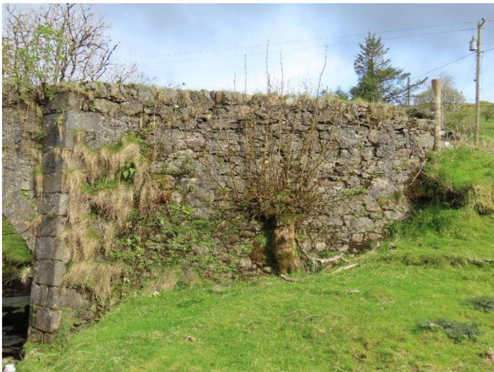
Photo 4 – stump of sycamore tree growing close to upstream bridge wall
