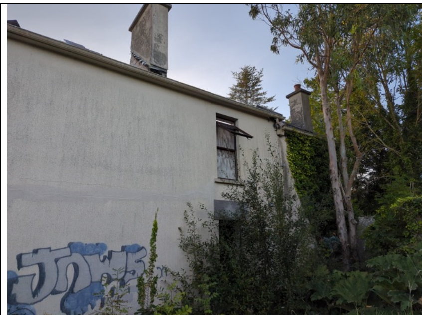
Plate 3. Eastern gable. Windows open and roof generally absent., Some ivy growth but not dense. Eucalyptus and willow in close proximity.
