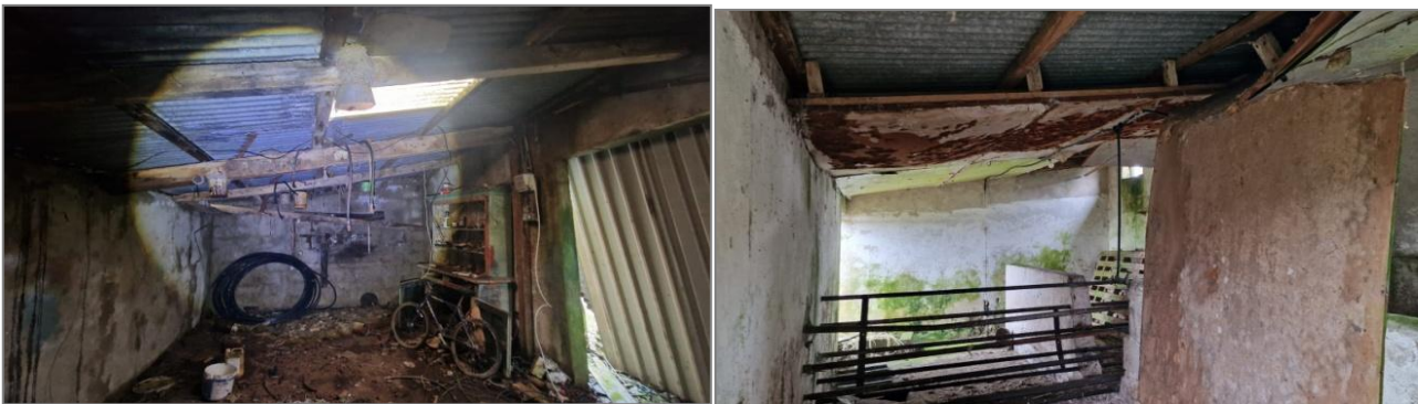
Plate 7. Part of outhouse with corrugated metal sheeting roof and ingress of daylight
