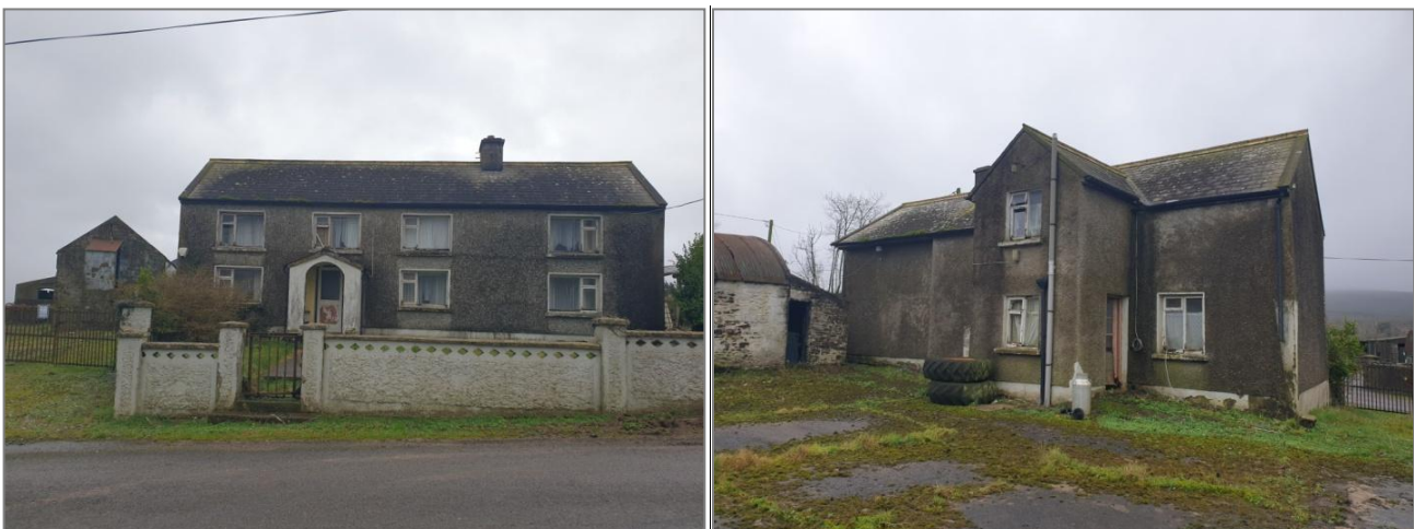
Plate 1. Photographs of the exterior of farmhouse proposed for renovation
