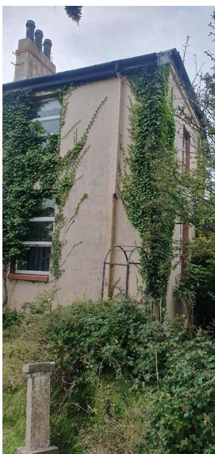
Figure 1. Corner of house with ivy cover where NPWS and KCC confirmed a bat roost
