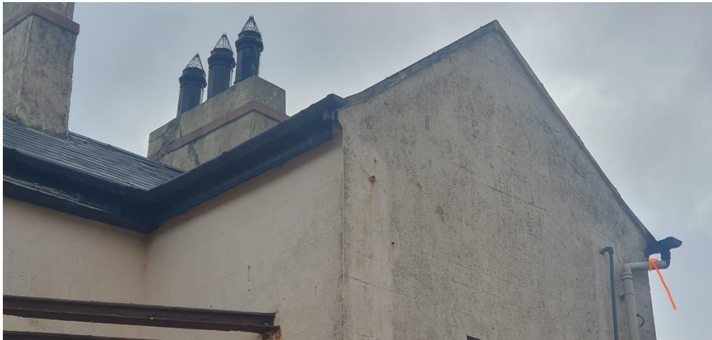
Figure 7. View of rear of the house, arrow indicates bat roost entrance
