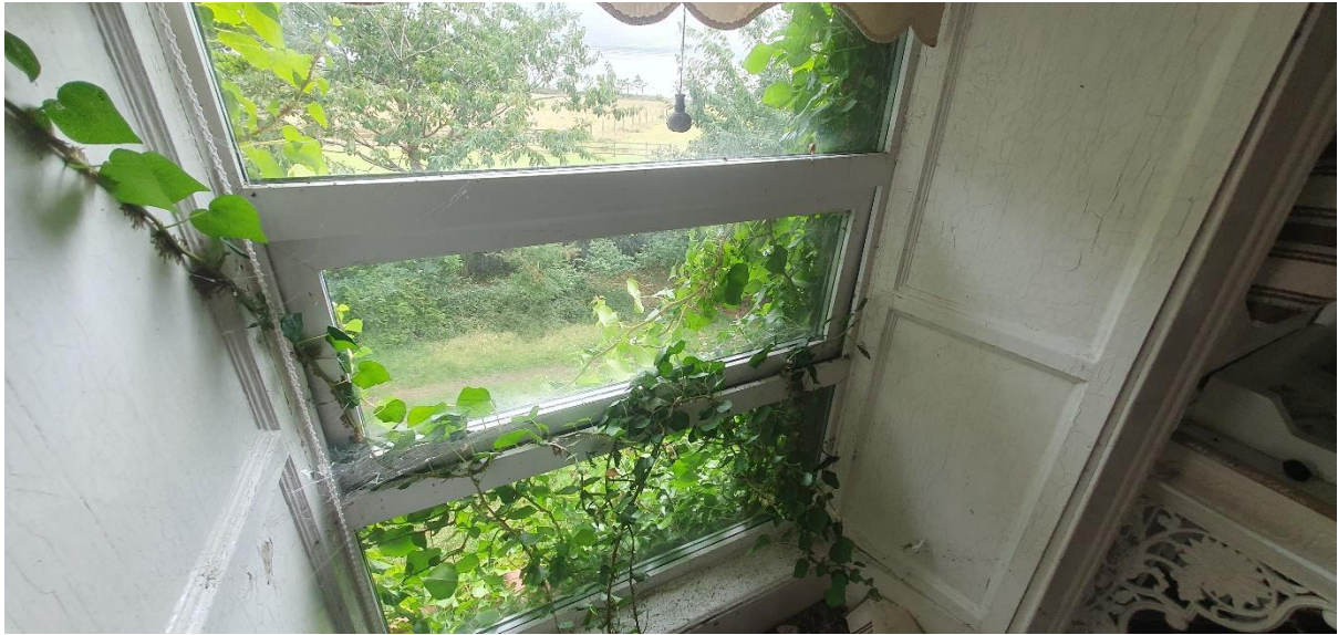
Photo 4. Ivy growing between window and window frame, but no gap for bats to enter first floor of the house
