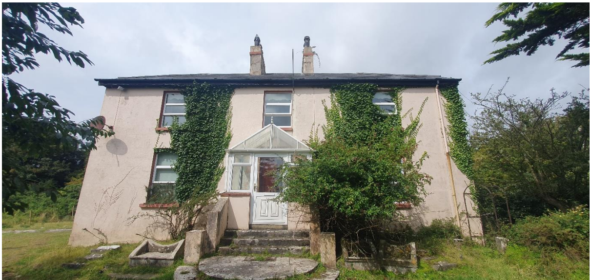
Photo 5. Front elevation of house to be demolished with significant ivy growth
