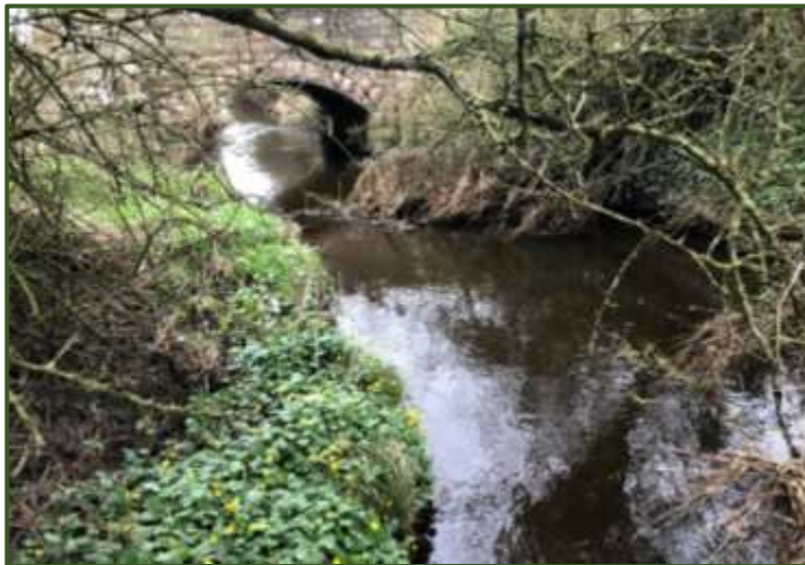
Picture 3: Image showing location of Lissanode Bridge prior to Bat Emergence Survey on 16/05/2024 – the infrared camera was positioned at this aspect
