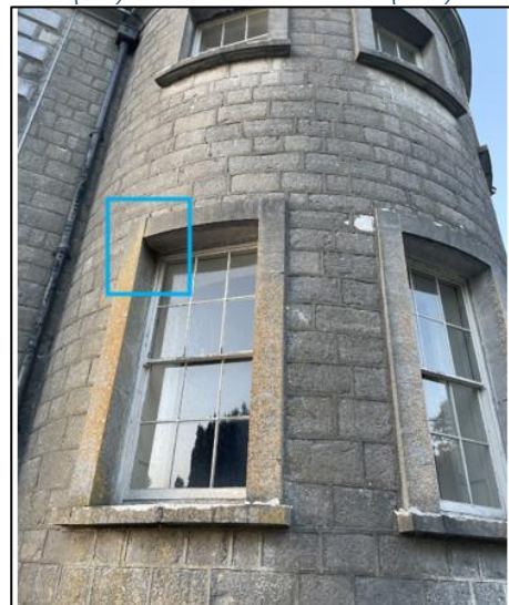
Plate 3 Bats recorded emerging from window crevice.
