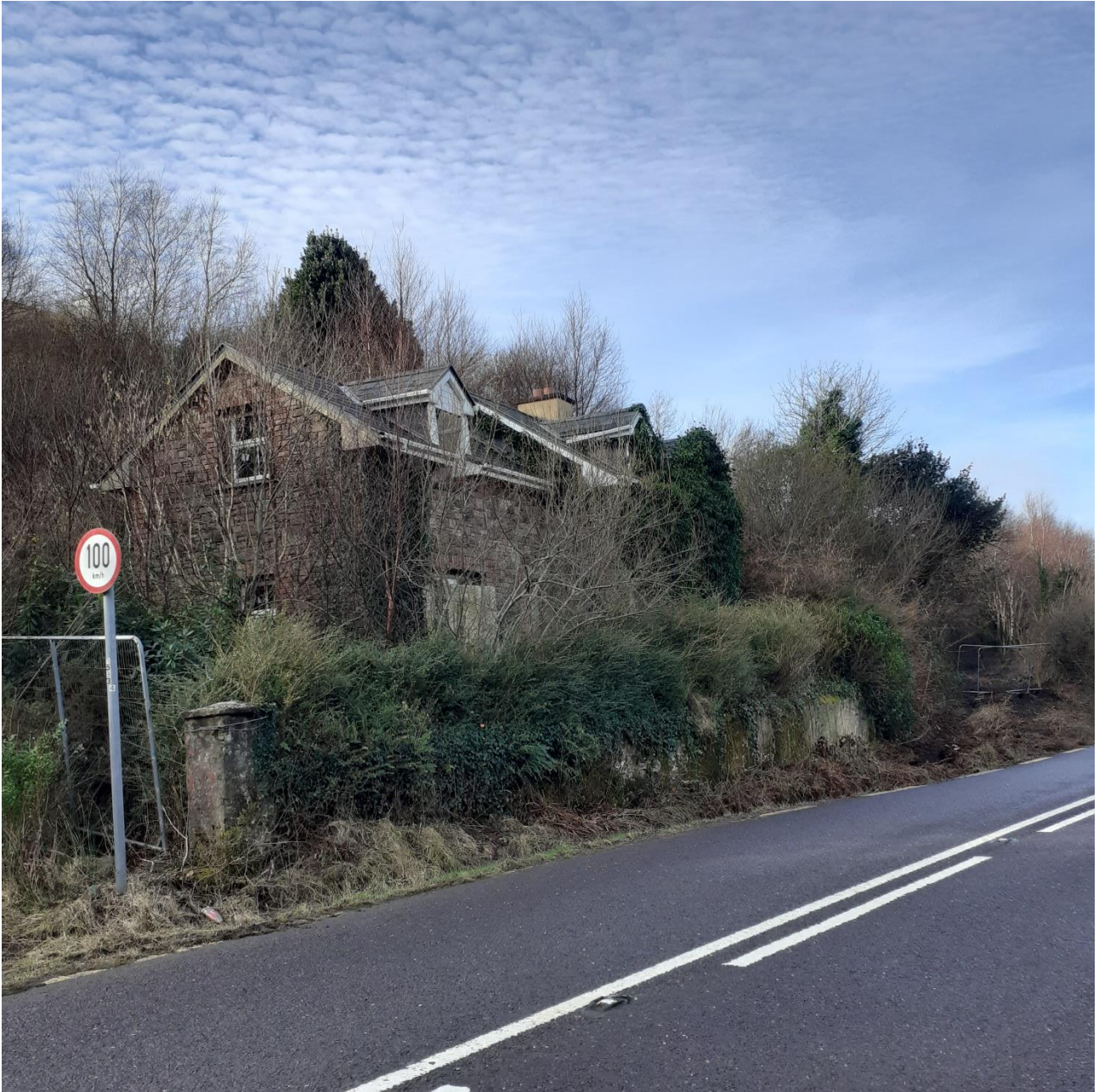
Plate 8: Wall and vegetation currently in place of the cottage.
