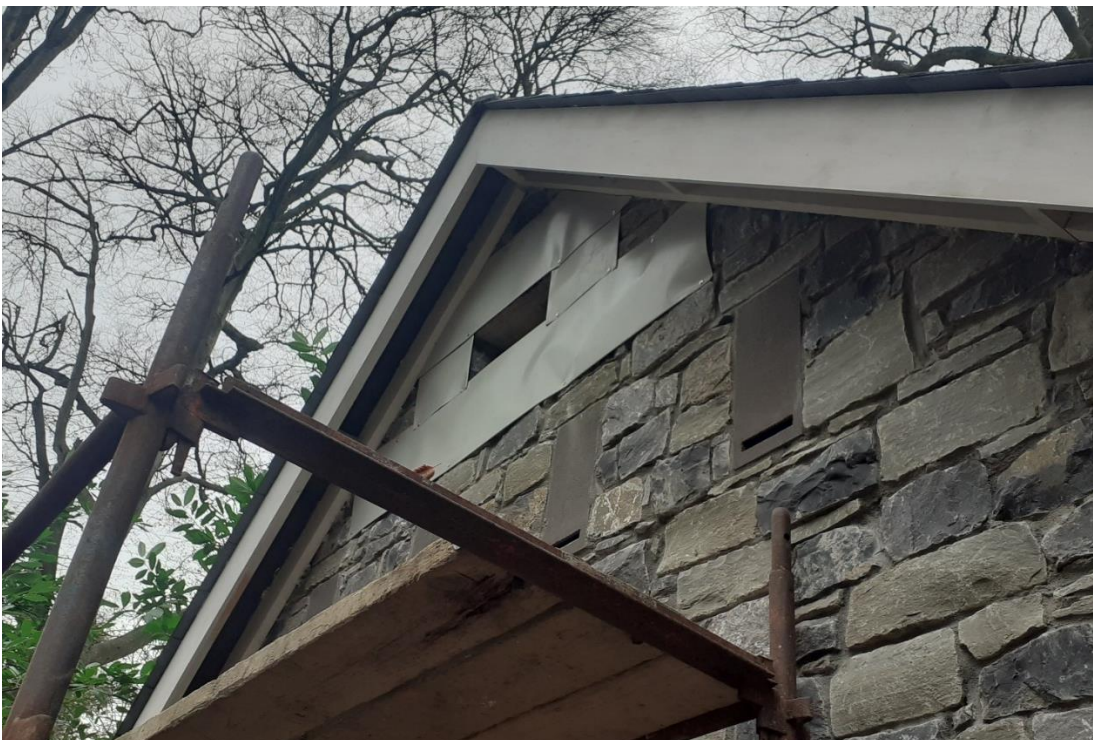
Plate 5b: Predator proofing on external wall around entrance point.
