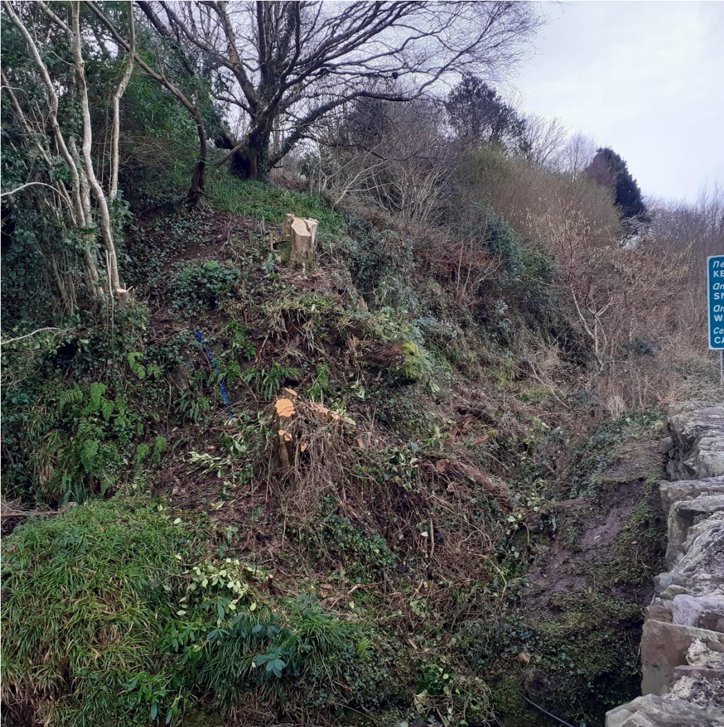
Plate 4: Blue line marks the proposed area of soil removal west of the existing bridge.
