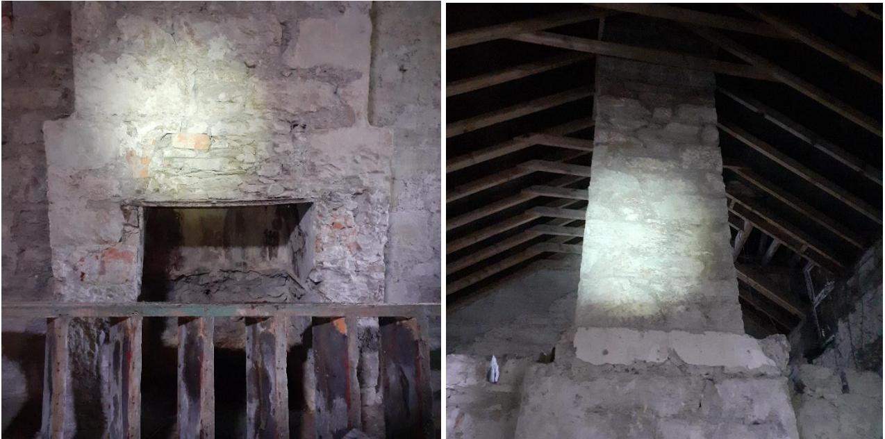
Plate 3a,b: Chimney structure inside the cottage.
