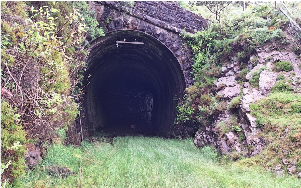
Plate 4 – Photograph of Drung Hill Tunnels (View west to westernmost tunnel).
