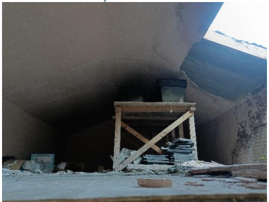
Plate 3-5 Converted and exposed attic.
