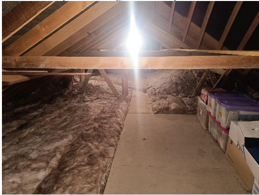
Plate 3-9 Illuminated, insulated attic.
