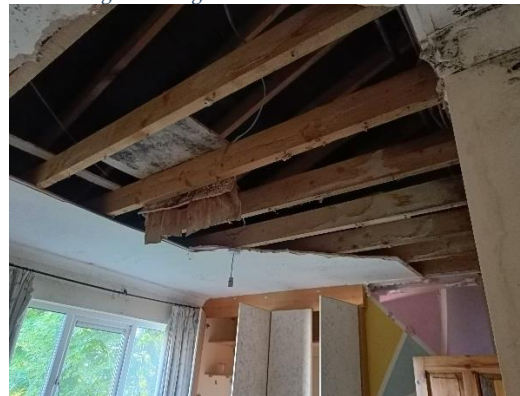
Plate 3-6 Access between first floor and attic.
