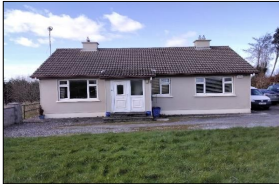
Plate 7 Bungalow for demolition with single attic space and two chimneys.
