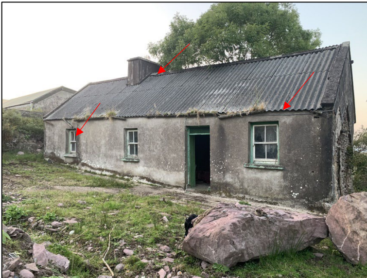
Plate 3-2: Suitable entry/exit points for bats in the disused dwelling at Treanmanagh
