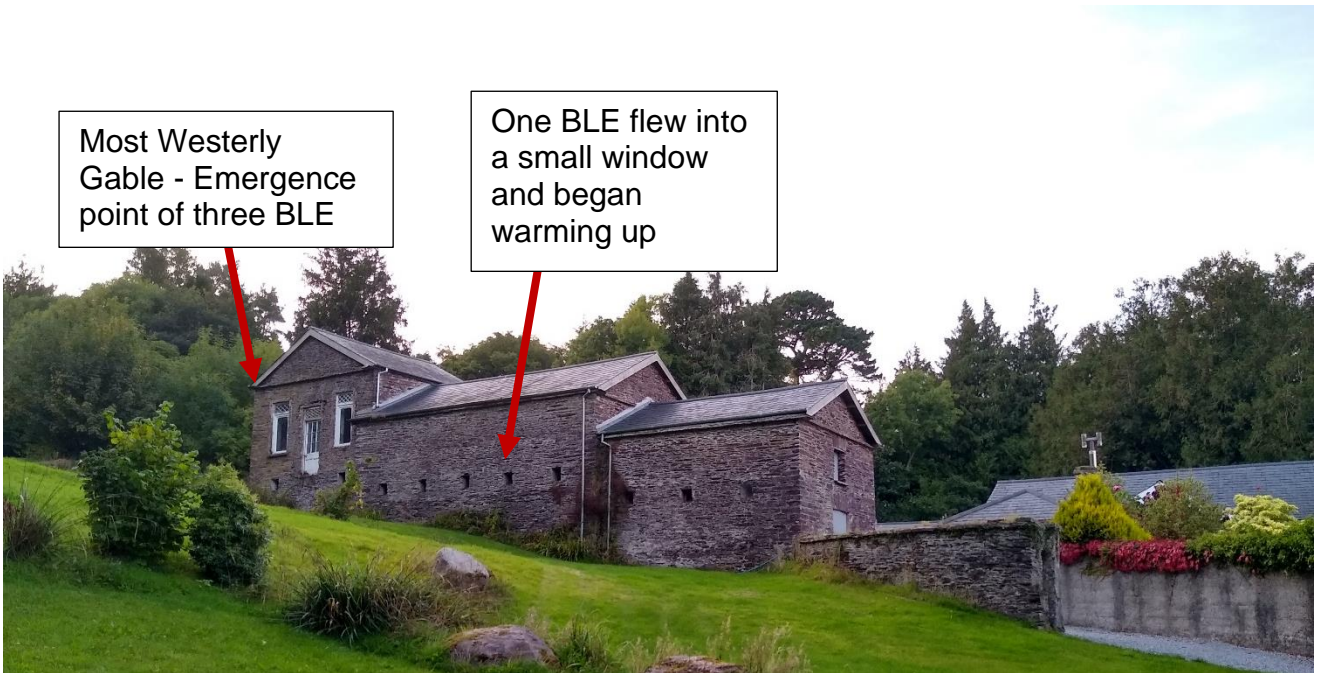
Figure 3-15: Rear of Stable building.
