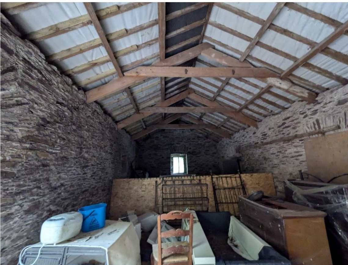
Figure 3-8: Interior photograph of second floor of agricultural store building.
