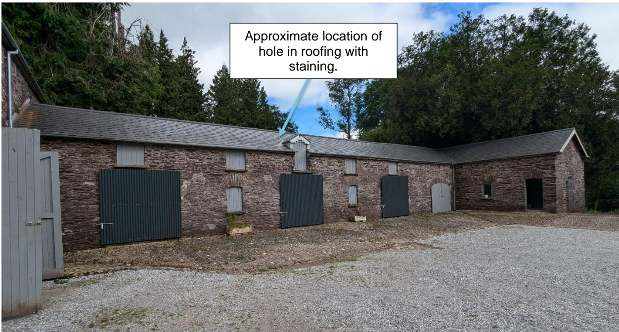
Figure 3-5: Cow byre building.
