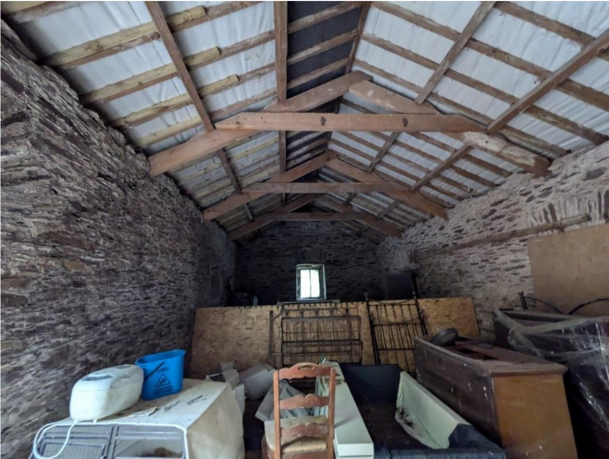
Figure 3-5: Interior photograph of second floor of 'Jam/Wine Cellar' building.
