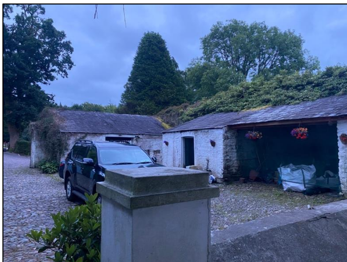
Plate 5 Outbuildings on the proposed development site.
