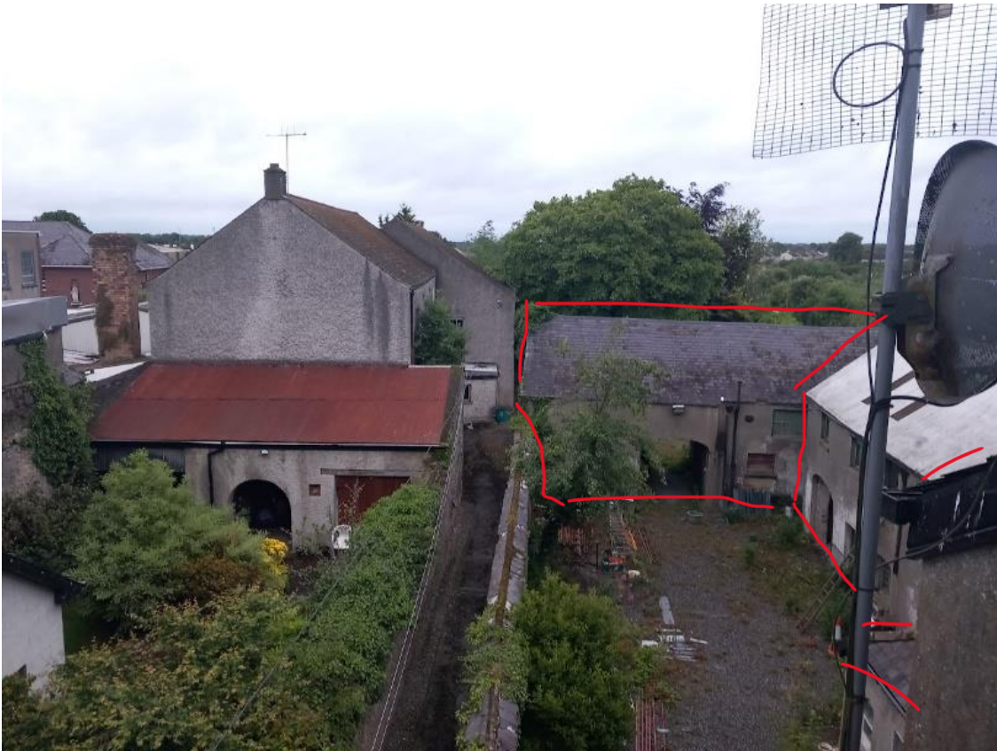
Figure 3-3 Two buildings for redevelopment
