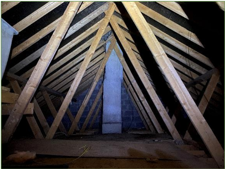
A2. Attic of residence.
