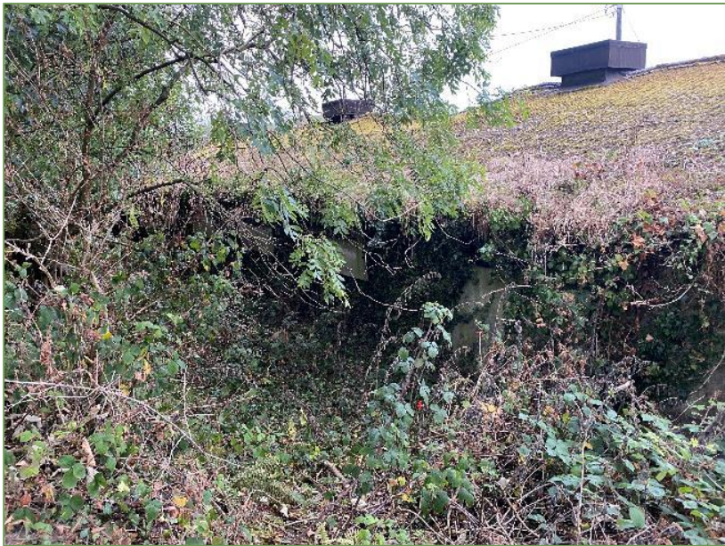
A5. Southern elevation of Hatchery 2.
