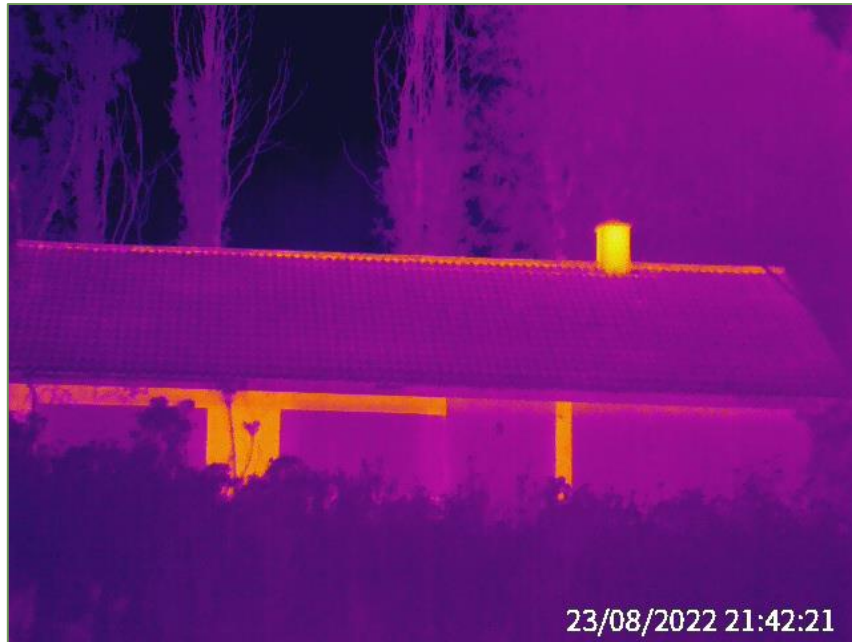
Plate 3.1 Example image from thermal camera covering western side of derelict residence.
