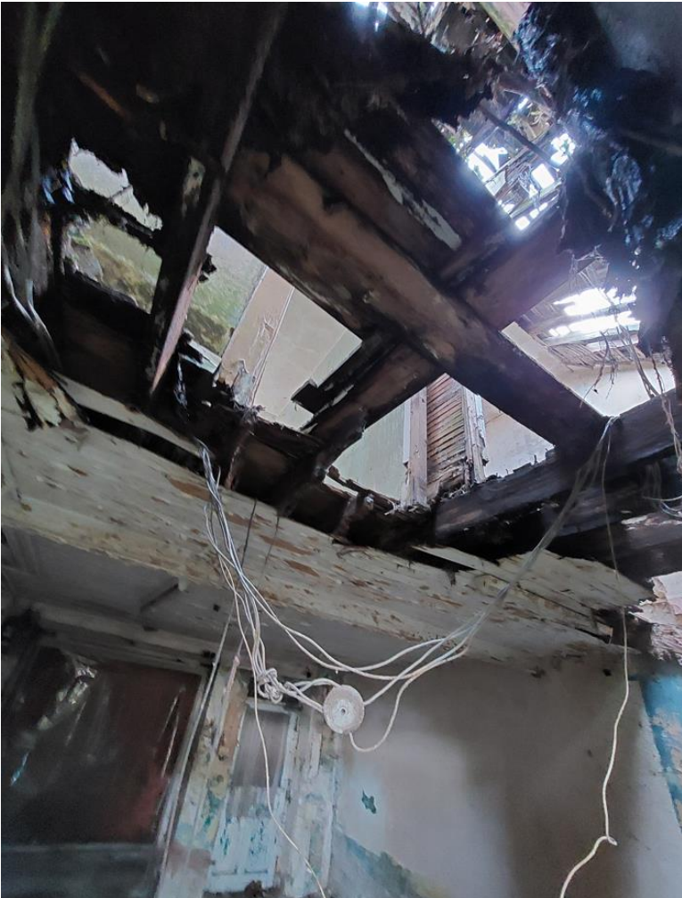
Photo 10: View from Ground floor looking up (first floor joists rotting and collapsed, roof structure rotting and collapsed in places. Not safe to access first floor. Area used for anti-social activity).
