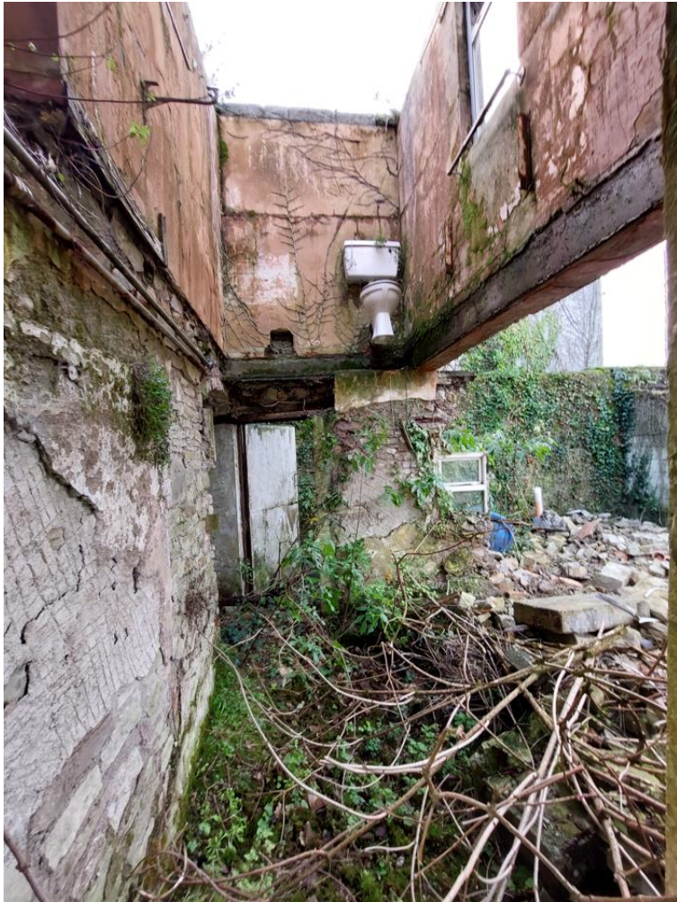
Photo 9: View of rear rooms (roof and first floor joists previously collapsed and removed).
