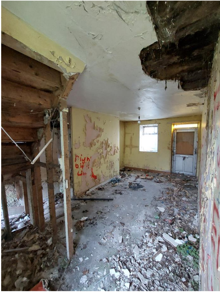
Photo 8: View from ground floor looking up (ceiling collapsing, first floor joists rotting)
