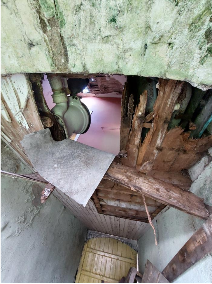
Photo's 6: View looking from ground floor up to first floor and roof (first floor joists and floors have rotten through and collapsed, roof structure rotting and collapsing in places. Not possible to safely access the first floor).
