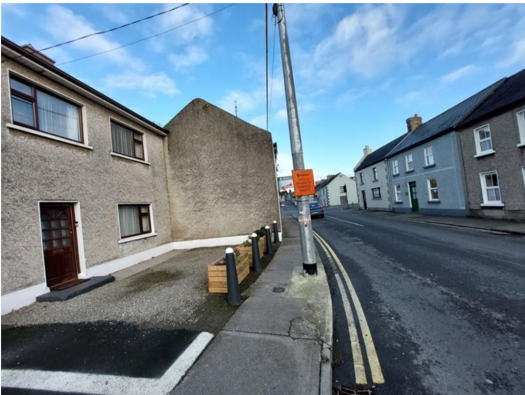
Photo 2: The existing houses are currently joined on the corner with a neighbouring property. This property is privately owned and occupied. This corner shows evidence of cracking, both building appear to be pulling away from each other. The more dilapidated the existing derelict structure becomes will have a direct affect on the private house. The proposed new development separates the new terrace houses from the private house. The new houses will also be set back in line with the front of this private house. This will provide a safer footpath, better visibility at the traffic lit junction and better stability for the private house.
