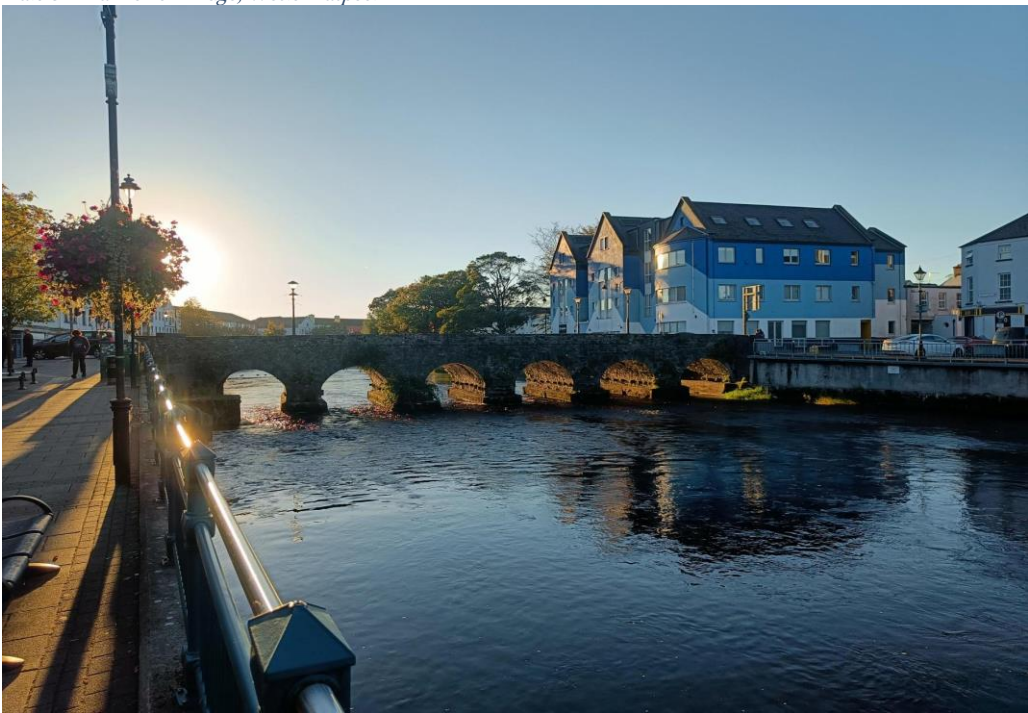
Plate 3-2 Markievicz Bridge; Eastern aspect
