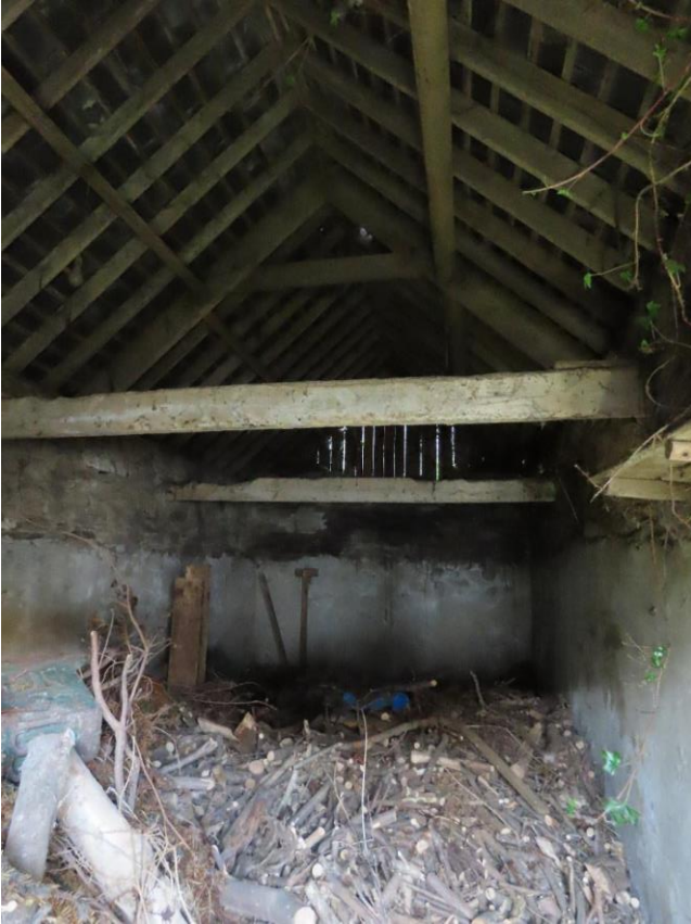
Photo 25 – interior of separate shed to south west of main outbuilding
