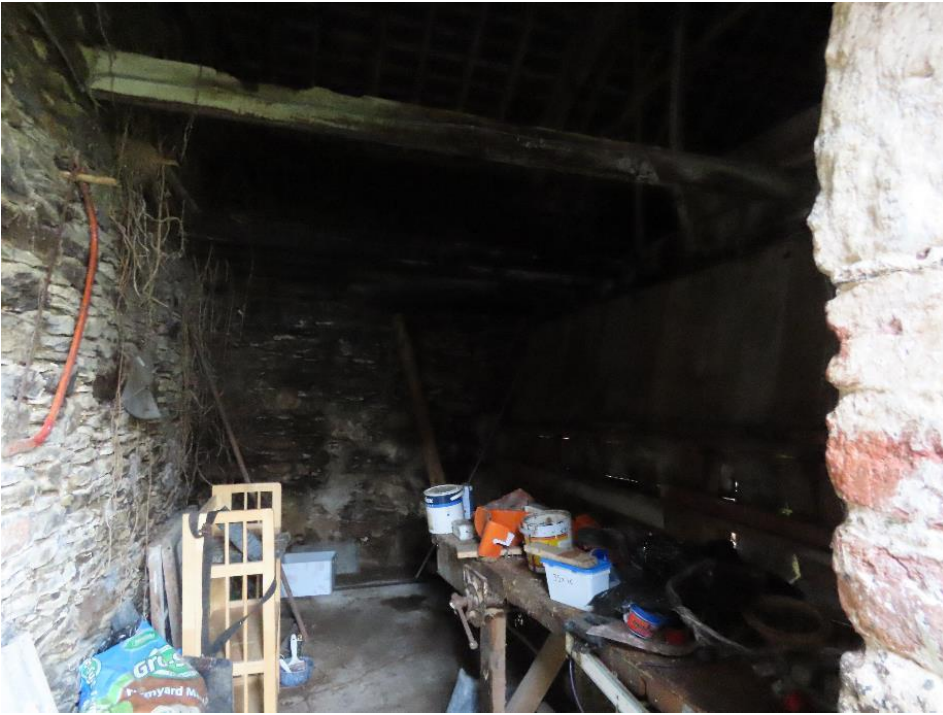
Photo 29 – workroom at south west end of long single storey outbuilding
