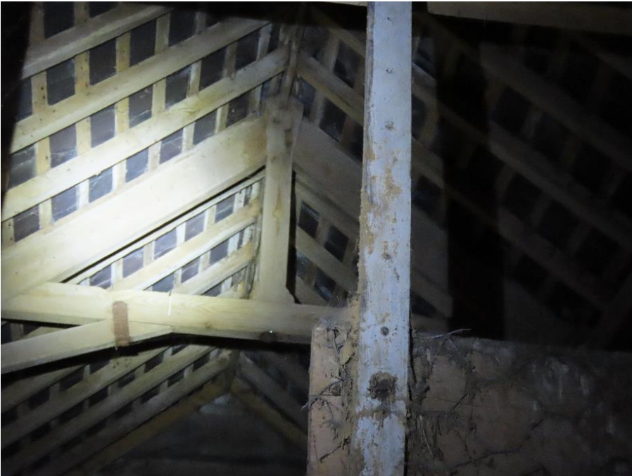
Photo 27– section of roof of long outbuilding above workroom
