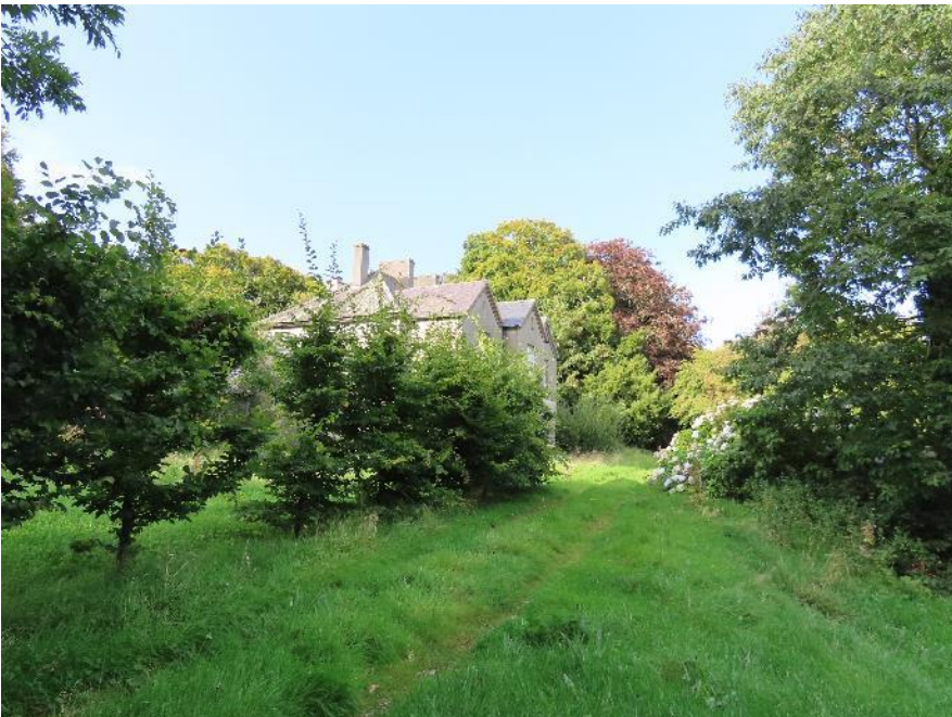
Photo 2 – south west corner of house showing setting of mature trees
