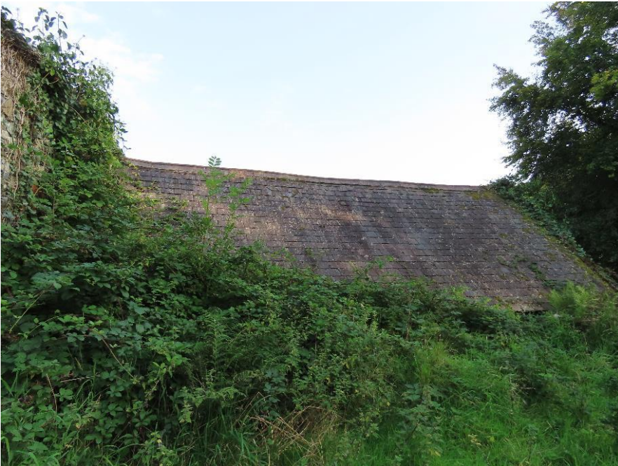
Photo 22 – Roof of single storey section of main outbuilding.
