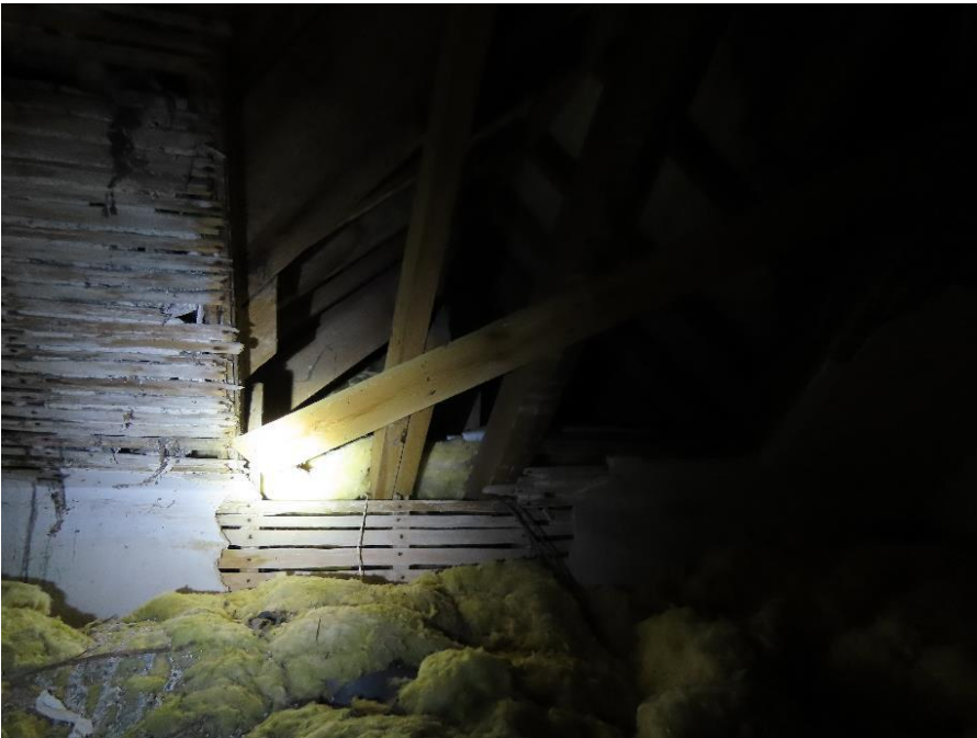
Photo 16 – main attic space
