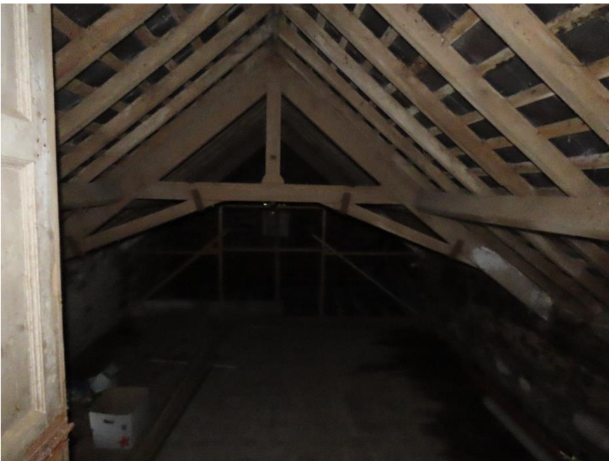
Photo 32 – view along length of attic space of long outbuilding
