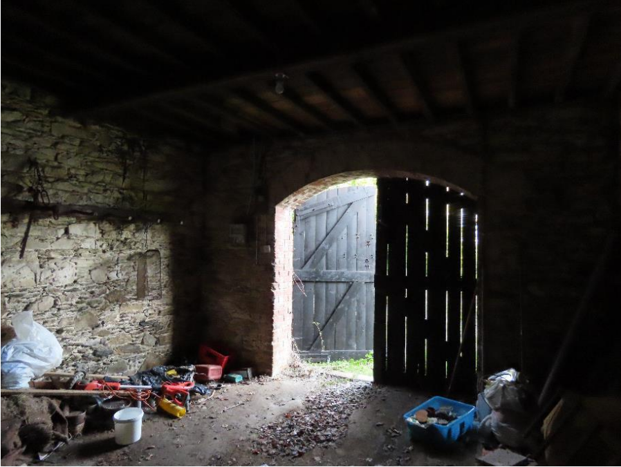
Photo 23 – ground floor of granary
