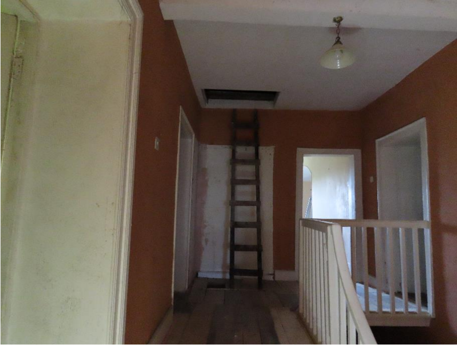
Photo 15 – access trapdoor to main attic on landing
