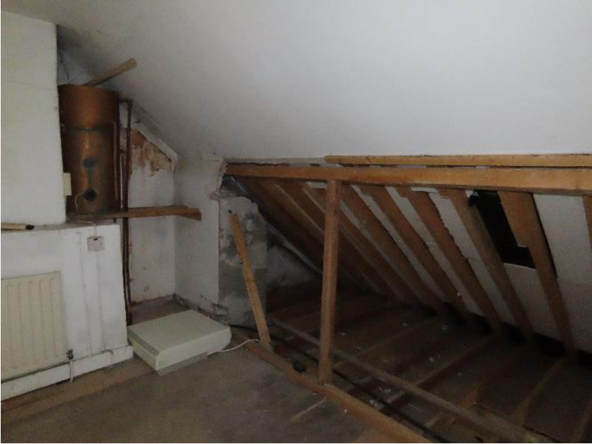
Photo 10 – exposed section of side roof in upstairs bathroom
