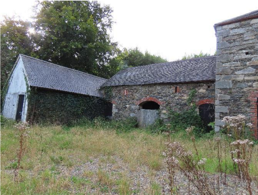
Photo 19 – long stone single storey building attached to granary
