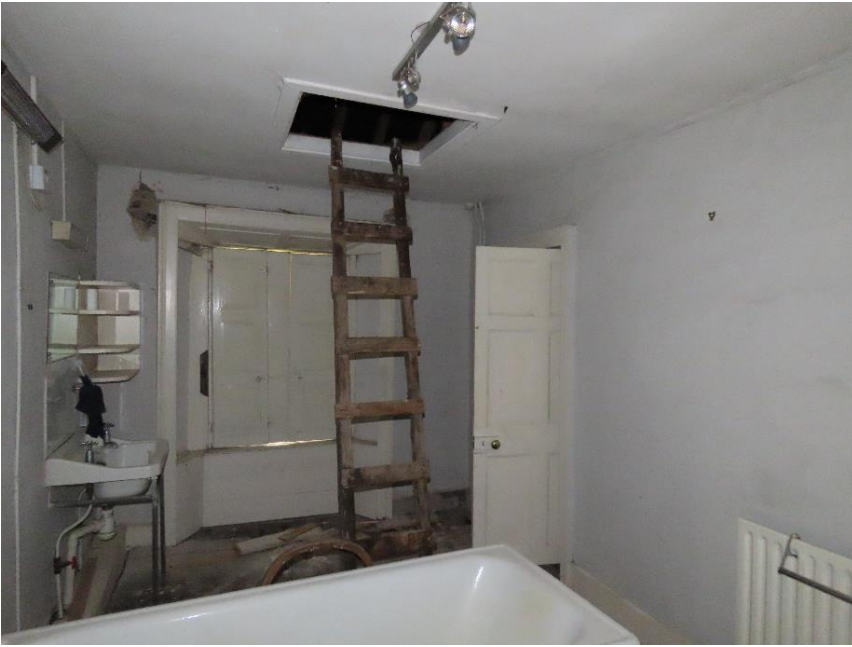
Photo 11 – access to attic space above bathroom
