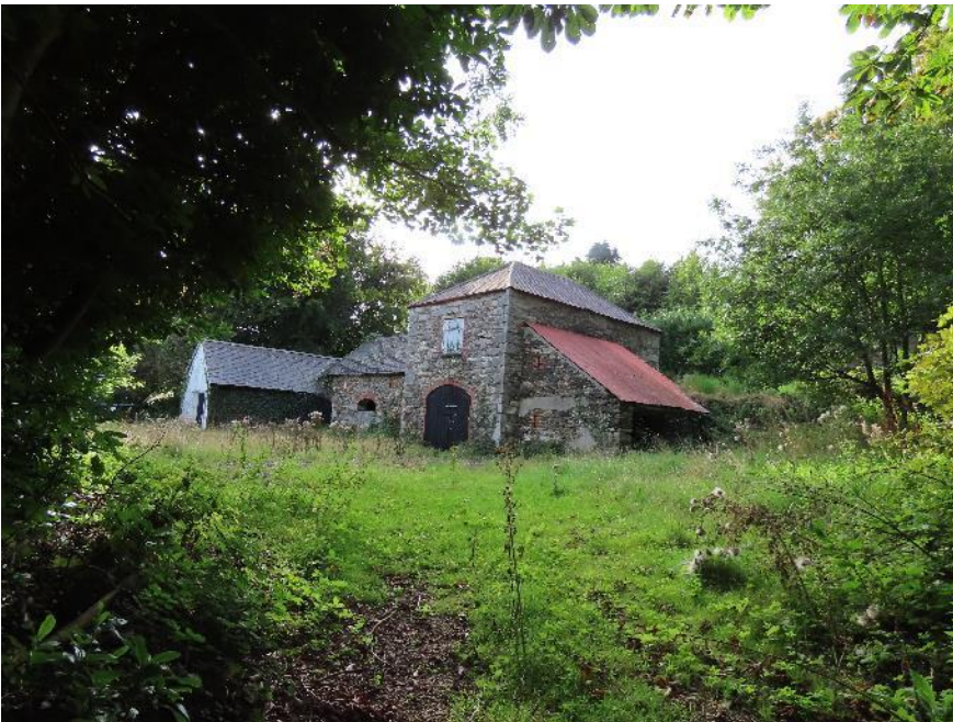
Photo 18 – main outbuilding showing two storey granary with stone lean-to
