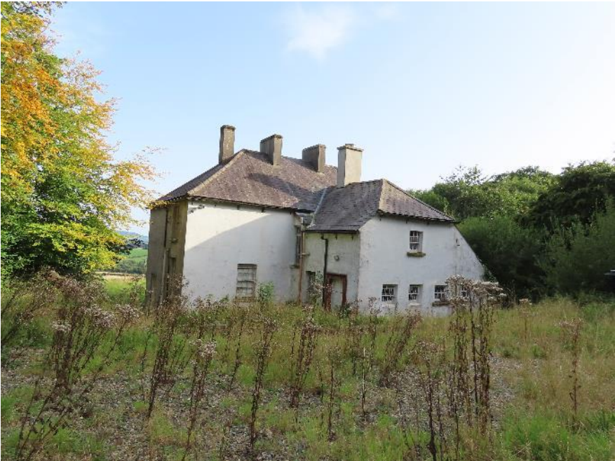
Photo 4 – rear of main house showing lower roofed section to rear
