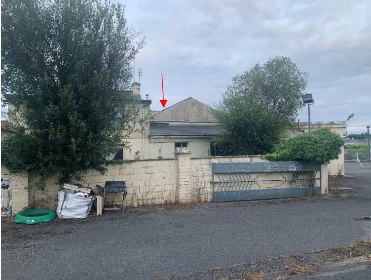
Plate 3-5: Raised section of roofing
