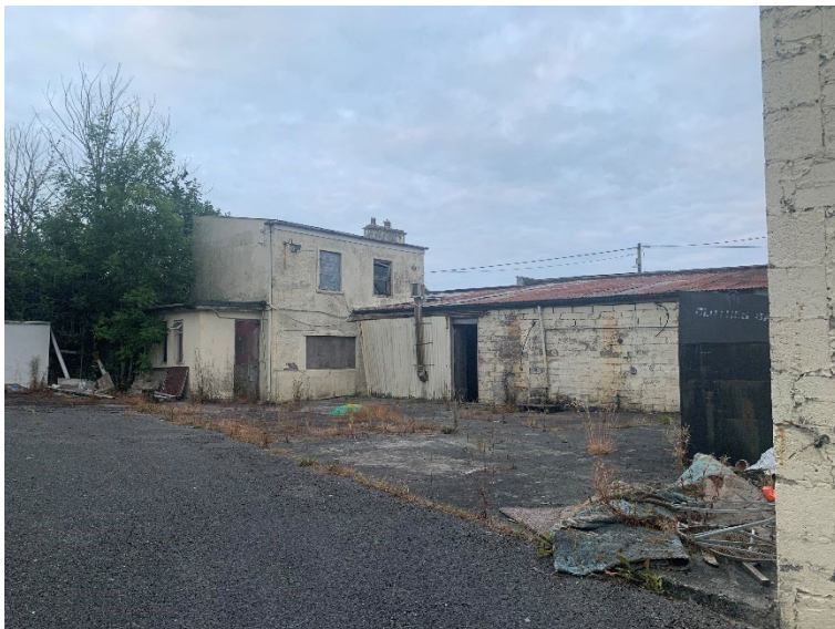
Plate 3-4: Workshop and 2-storey building
