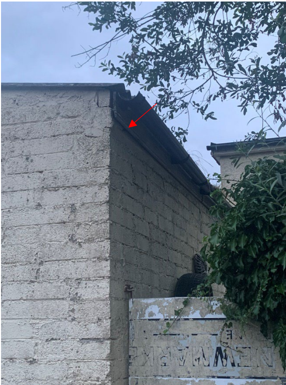
Plate 3-8: Raised fascia board
