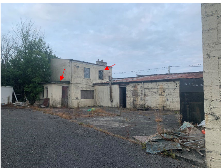
Plate 3-9: Potential access points at fascia board and window
