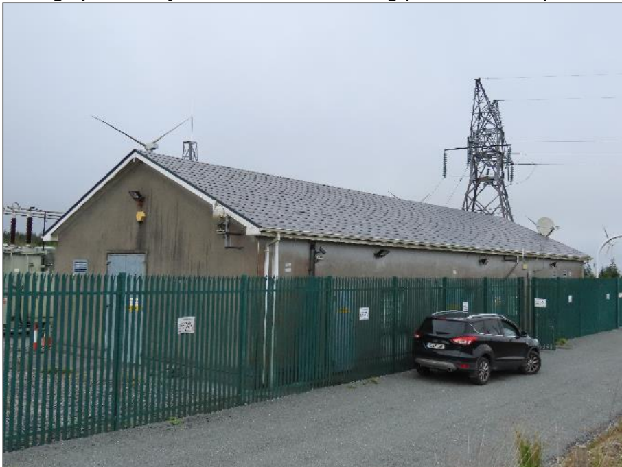
Photograph 2: Derrybrien Substation building (south elevation)
