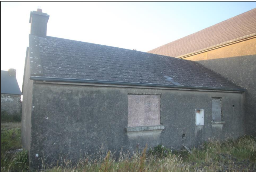
Plate 6 Other side of old extension, no missing slates/access on this side.
