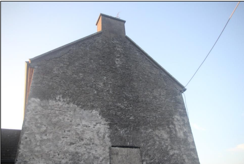
Plate 3 Side façade well sealed.
