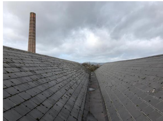
Plate 2 Central roof valley, intact slate work.
