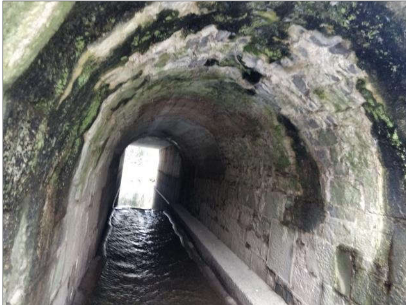
Plate 2.5 Lombardstown Bridge under the arch.
