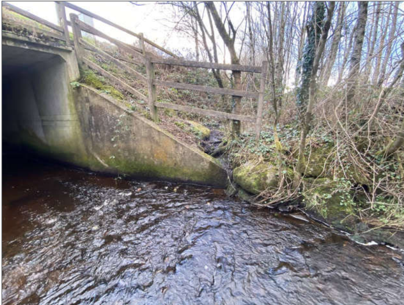
Plate 5.22b Small stream flowing over northern wingwall at Knockeennagowan Bridge.
