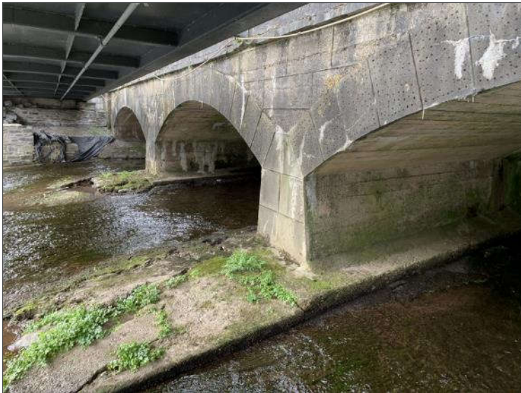
Plate 2.1 Killeagh River Bridge.
