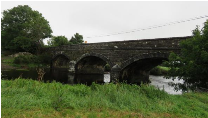
Photo 1 – Duncannon Bridge – large bridge with 3 arches spanning the River Blackwater
