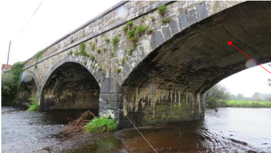
Photo 2 – Duncannon Bridge – showing some shuttered grouting under eastern arch
