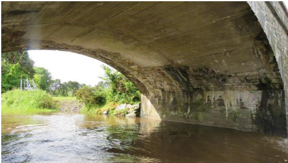
Easternmost arch – shutter cement applied to arch apex
