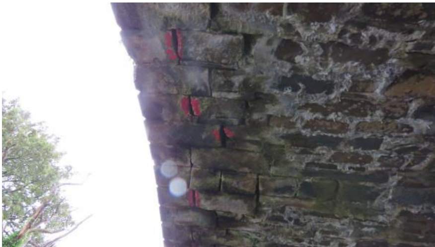
Photo 5 – Duncannon Bridge – 4 crevices marked for retention behind facing stones
