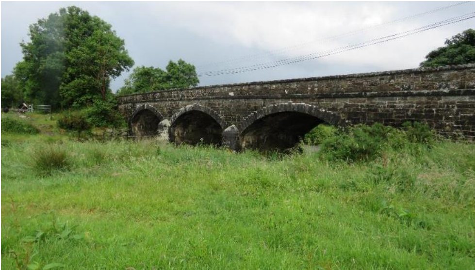
Upstream elevation of Duncannon Bridge
