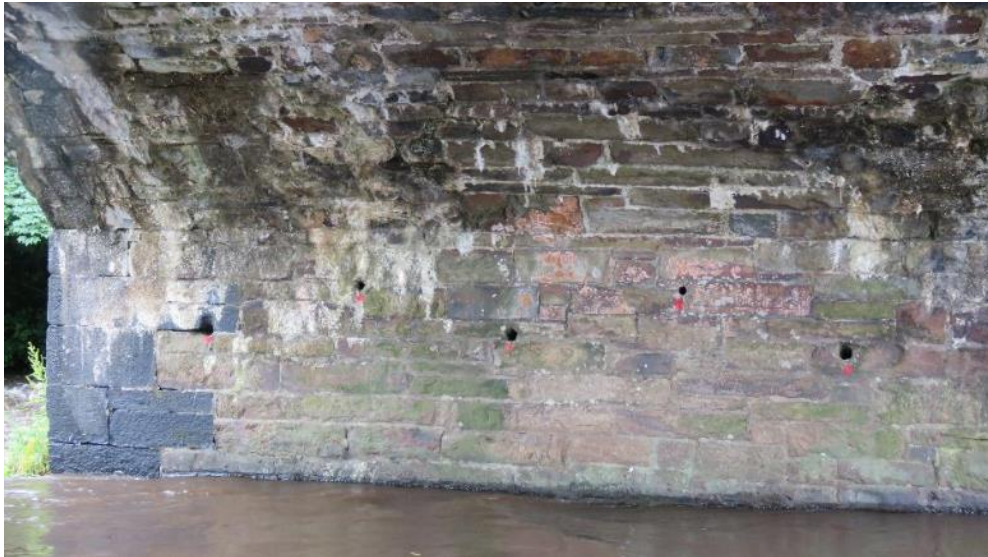
Series of 5 bore holes under the western arch – all occupied by nesting sand martins
