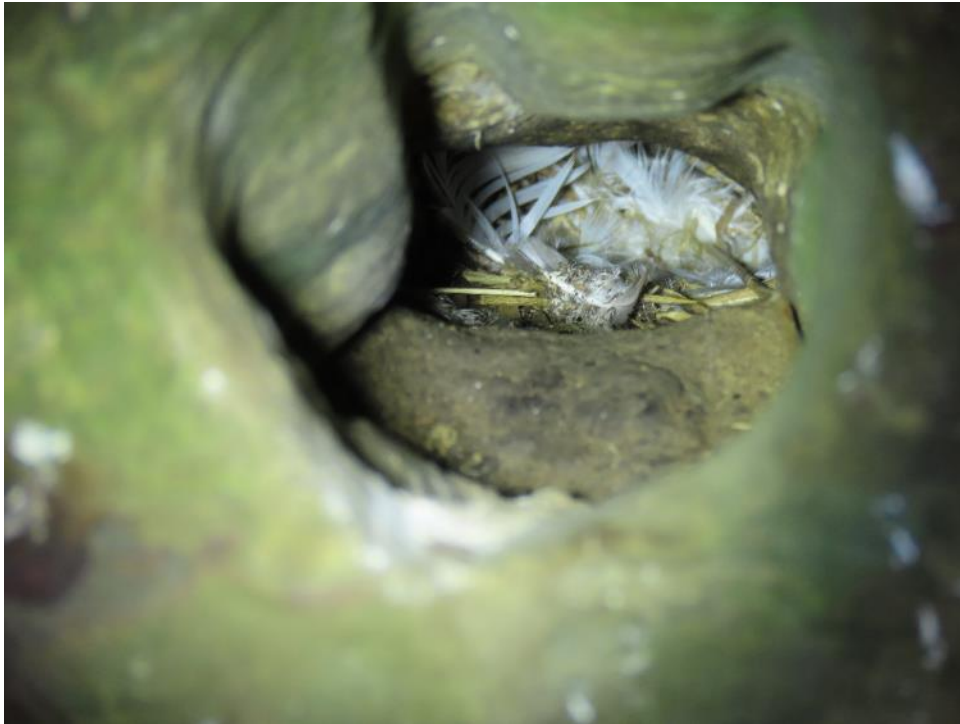
Duncannon Bridge – sand martin nest in borehole in abutment
