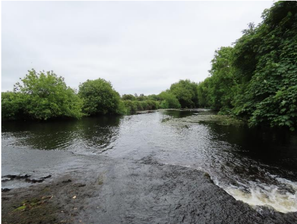
Duncannon Bridge – view of watercourse downstream
