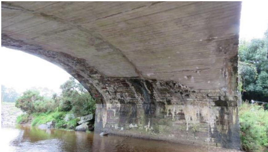
Photo 3 – Duncannon Bridge – close-up of shuttered grouting under eastern arch
