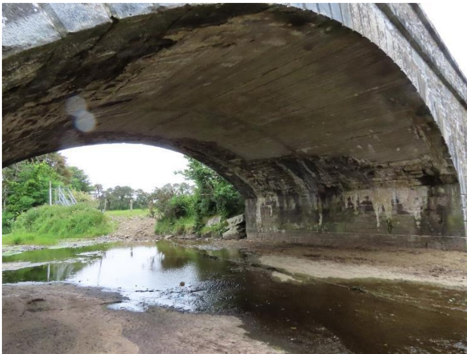
Duncannon Bridge – easternmost arch
