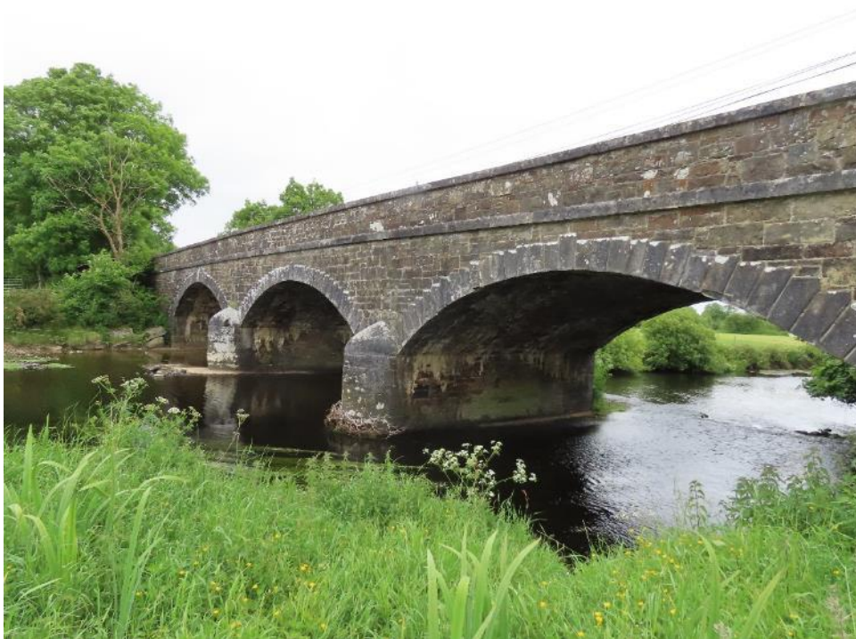
Duncannon Bridge – upstream elevation
