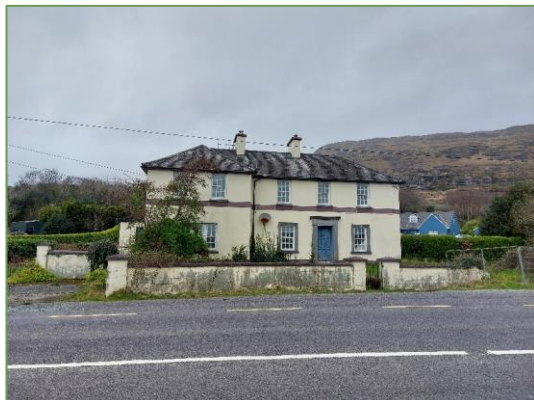
Plate 3.2.1 View overlooking the front aspect of the former Garda Station.
