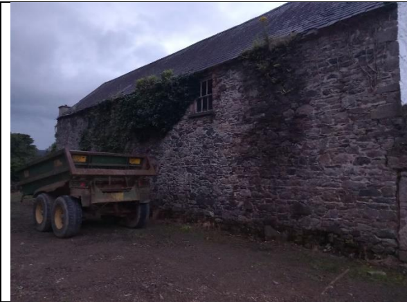
Northern exterior of stable B
