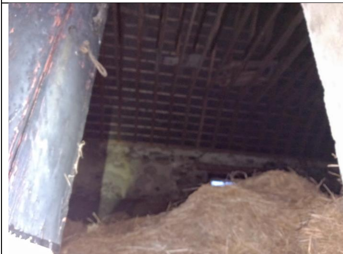
Interior of loft space Stable B
