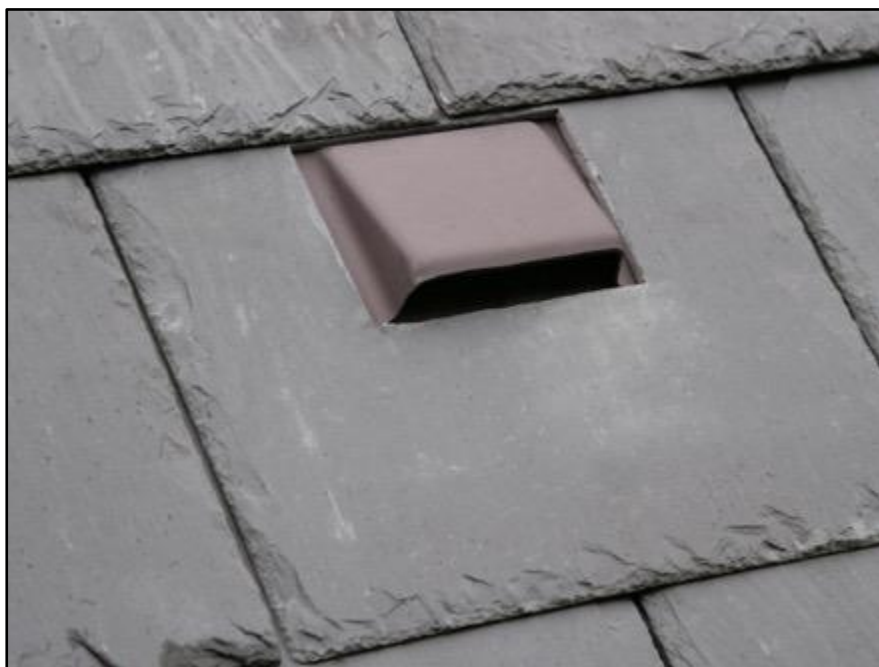
Figure 7. Example of an adapted roof slate that permits bat access to a roof space.
